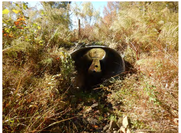
Dry Creek Reach 4 – Looking Downstream (10/18/2022)
