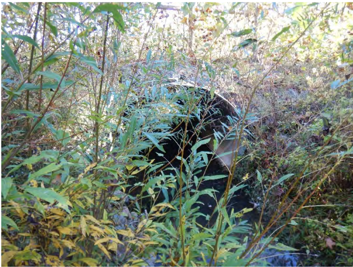
Dry Creek Reach 2 – Looking Upstream (10/18/2022)
