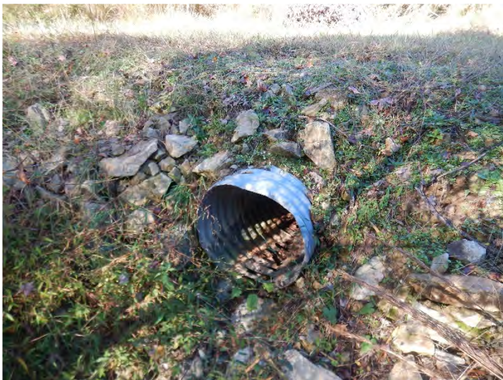
UT5 – Looking Upstream (10/18/2022)
