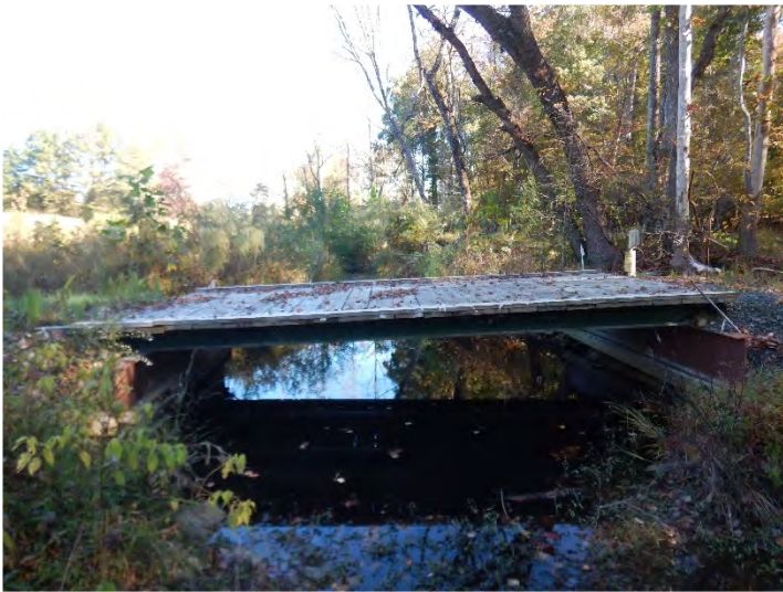
Dry Creek Reach 2 – Looking Upstream (10/18/2022)
