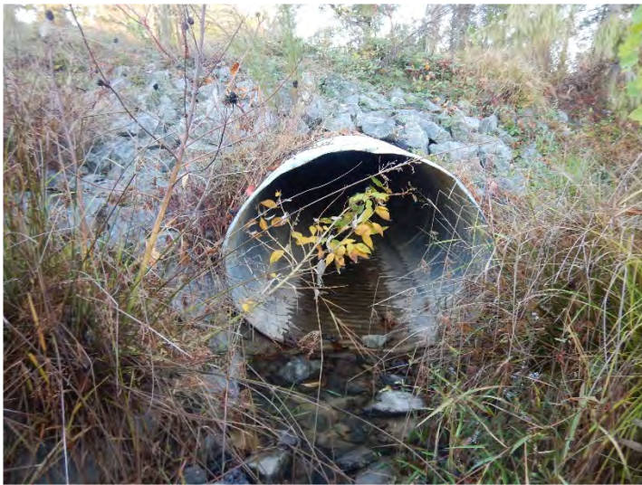
UT1 Reach 2 – Looking Upstream (10/18/2022)
