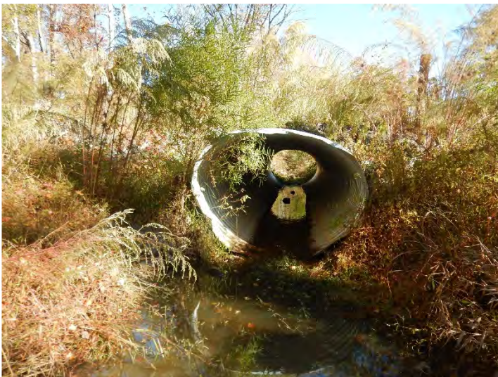
Dry Creek Reach 4 – Looking Upstream (10/18/2022)
