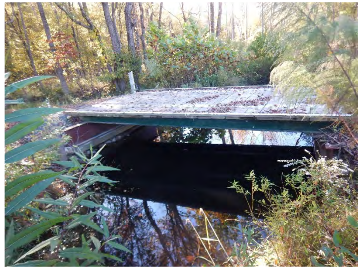
Dry Creek Reach 2 – Looking Downstream (10/18/2022)
