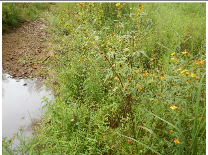
After – Repaired Localized Erosion (09/16/2021)
