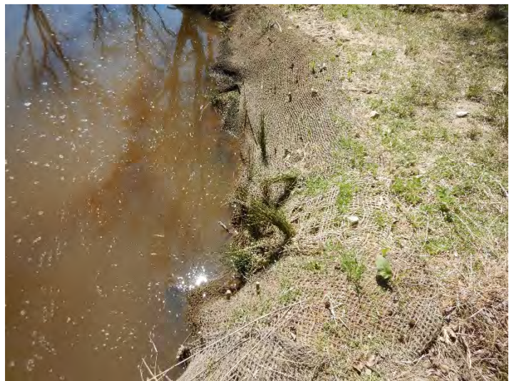
After – Repaired Localized Erosion (04/2/2021)
