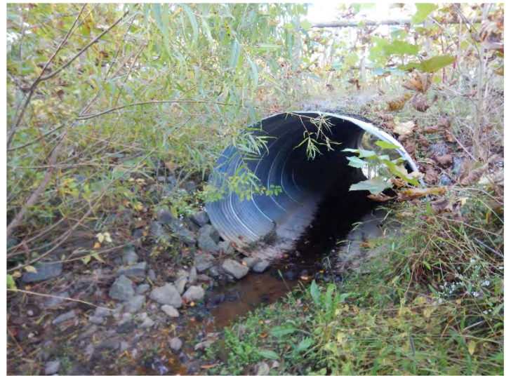
Dry Creek Reach 2 – Looking Downstream (10/18/2022)
