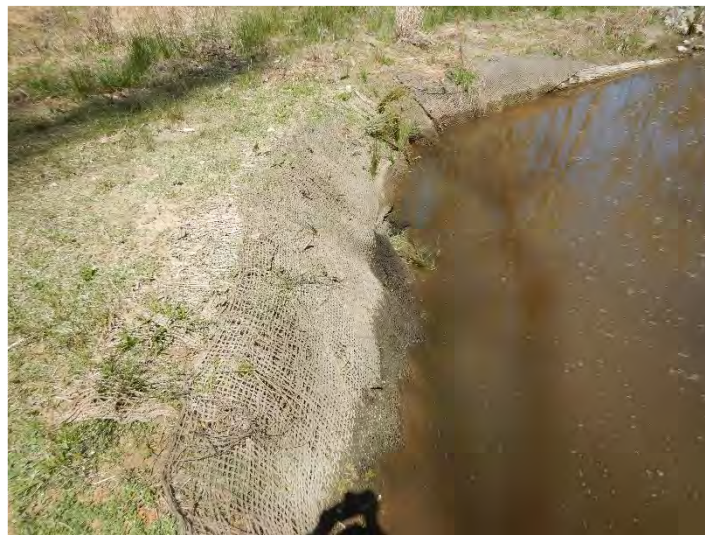
After – Repaired Localized Erosion (04/2/2021)
