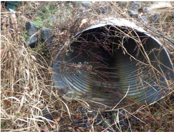
UT1 Reach 2 – Looking Upstream (12/7/2023)
