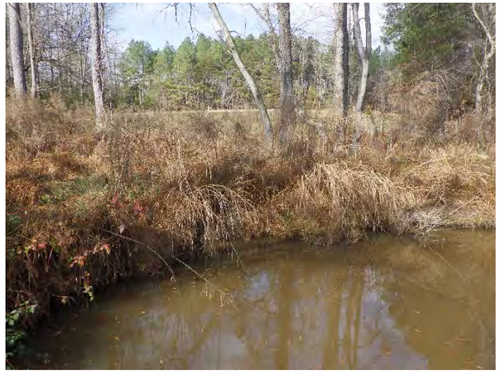
After – Repaired Localized Erosion (11/8/2023)
