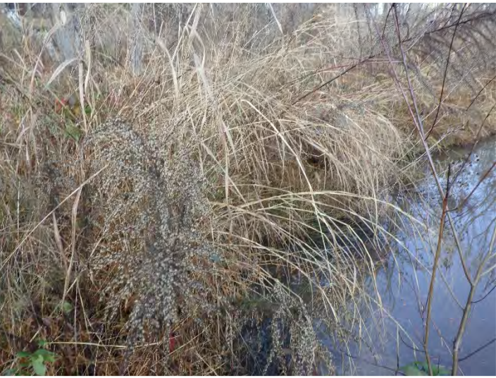
After – Repaired Localized Erosion (11/8/2023)
