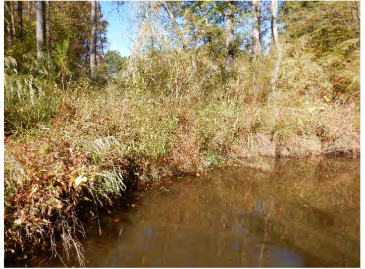
After – Repaired Localized Erosion (10/18/2022)
