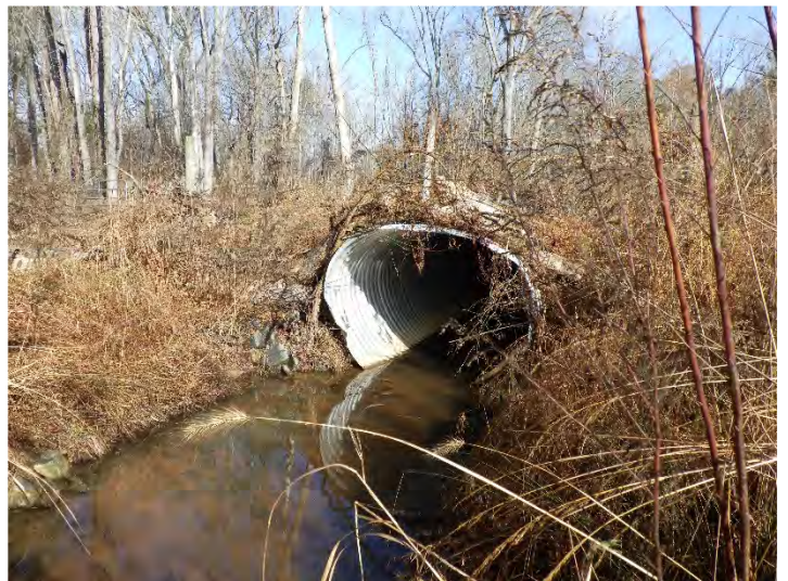
Dry Creek Reach 4 – Looking Downstream (12/7/2023)
