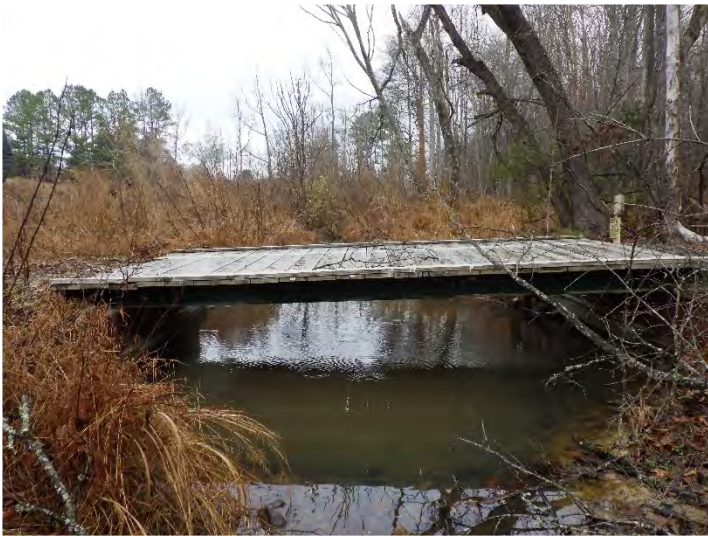
Dry Creek Reach 2 – Looking Upstream (12/7/2023)
