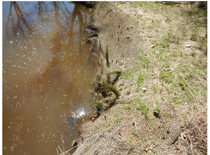
After – Repaired Localized Erosion (04/2/2021)
