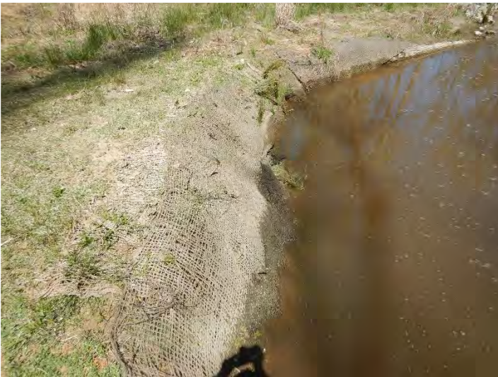
After – Repaired Localized Erosion (04/2/2021)
