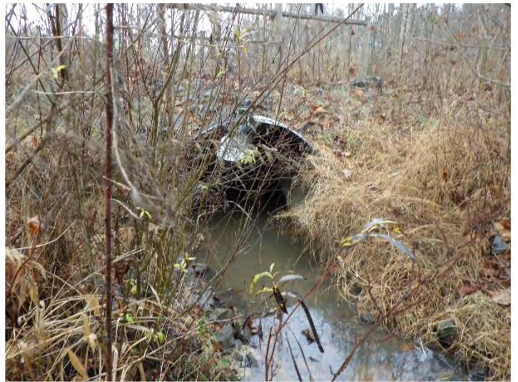
Dry Creek Reach 2 – Looking Downstream (12/7/2023)
