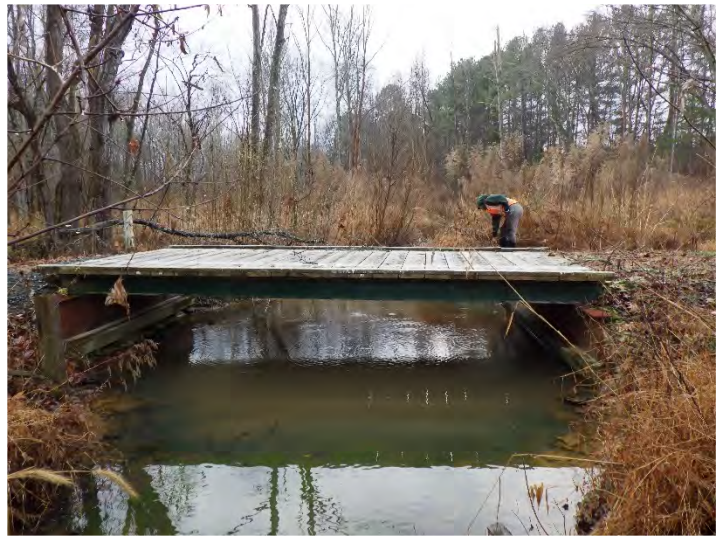
Dry Creek Reach 2 – Looking Downstream (12/7/2023)
