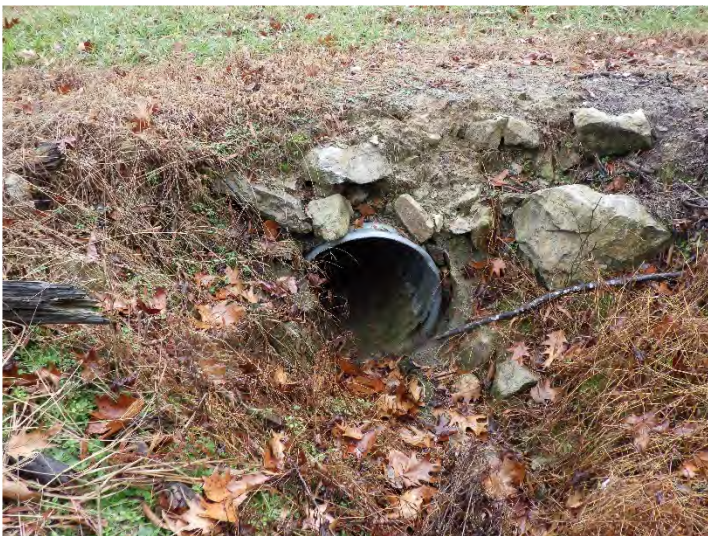
UT5 – Looking Upstream (12/7/2023)
