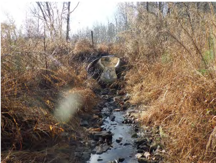
Dry Creek Reach 4 – Looking Upstream (12/7/2023)
