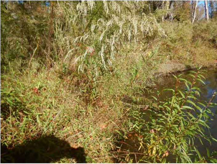
After – Repaired Localized Erosion (10/18/2022)
