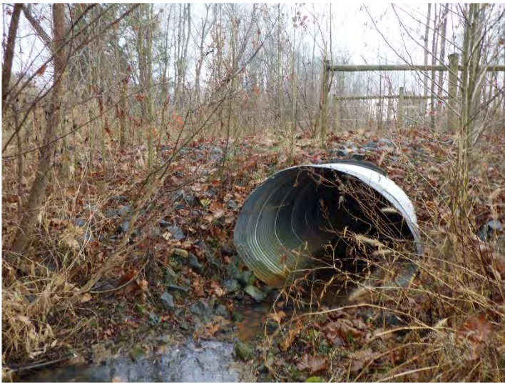
Dry Creek Reach 2 – Looking Upstream (12/7/2023)
