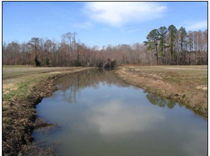
Looking downstream towards woodline at overly widened UT1 channel.
