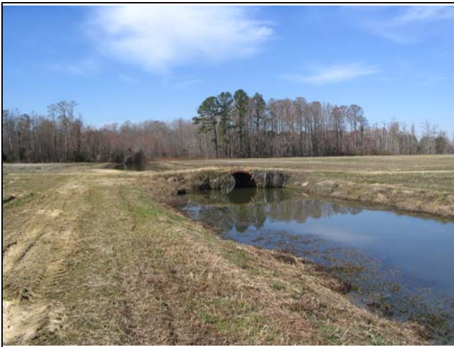
Existing UT1 culvert crossing along farm access road.
