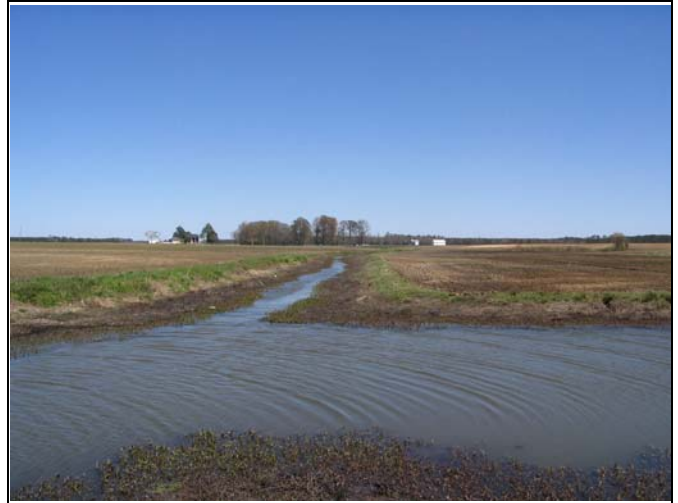
Looking upstream at Pond #3 tying into UT1 channel.
