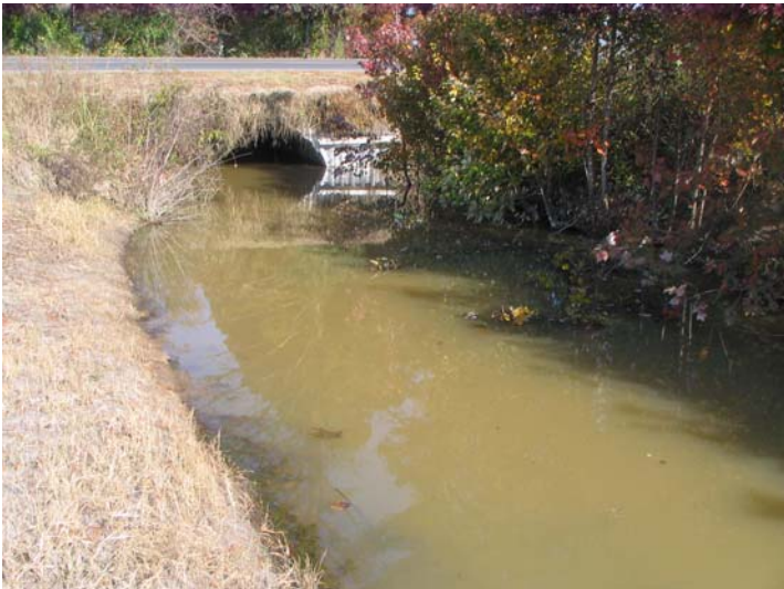
Upstream culvert crossing under Kellogg Fork Rd Station 10+00.JPG
