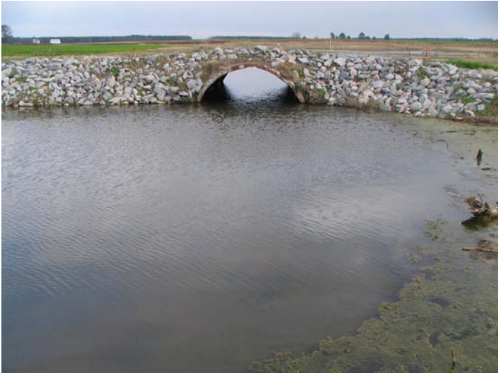
PP8 Downstream Culvert Crossing Station 44+50.JPG
