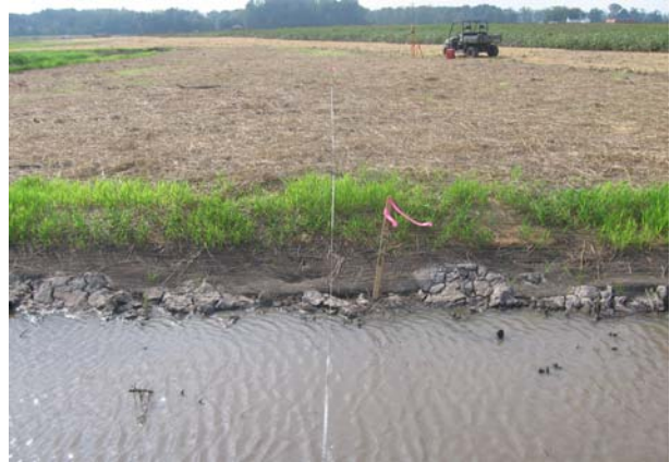
Looking at the Right Bank
