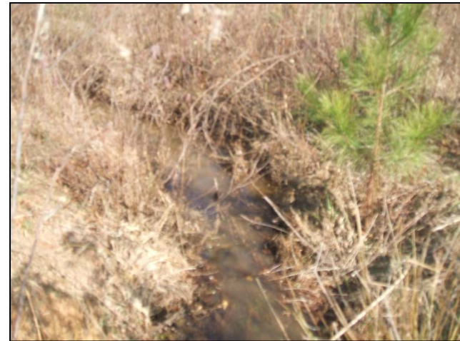
Cross-Section 2-View Downstream Tributary (1/2010)
