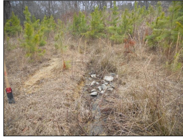
Cross-Section 3-View Downstream Tributary (2/2011)
