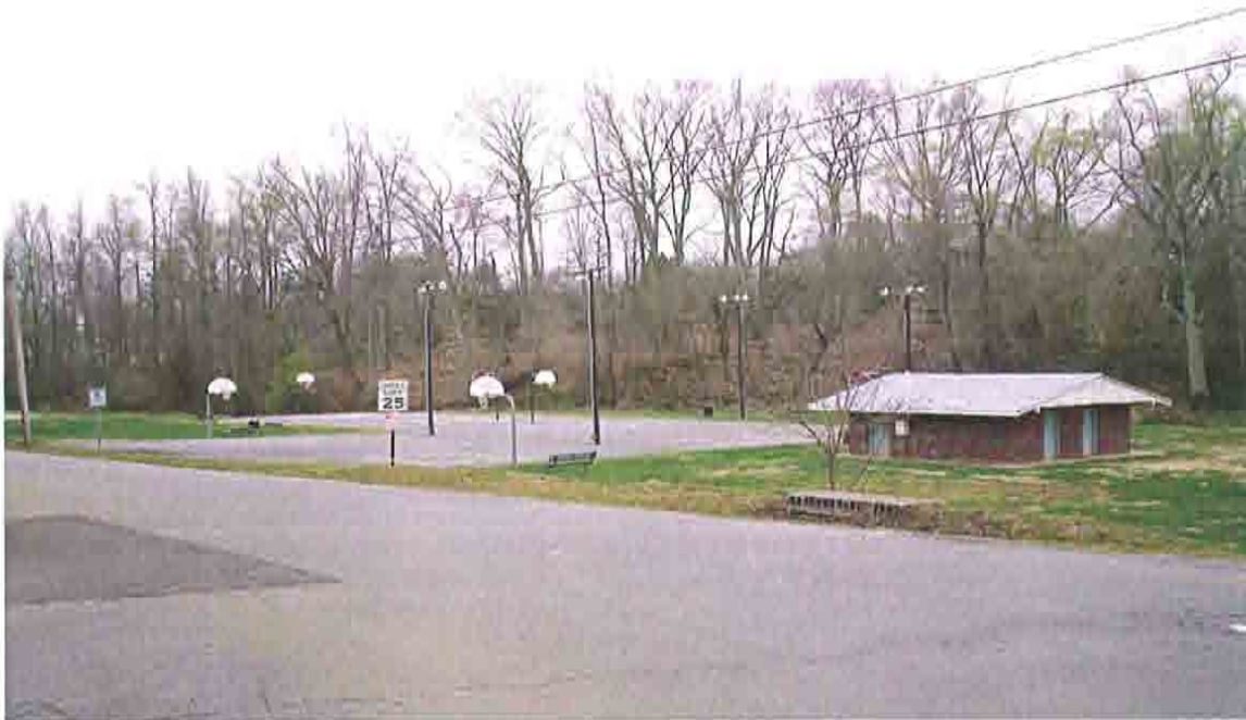
Existing basketball courts along middle reach of Dye Branch. Proposed area for channel relocation.
