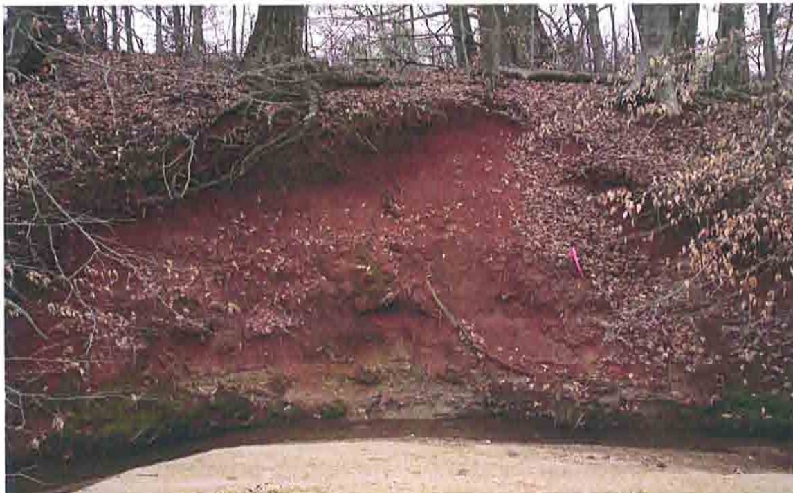
Eroded banks along western side of basketball courts. Dye Branch middle reach.
