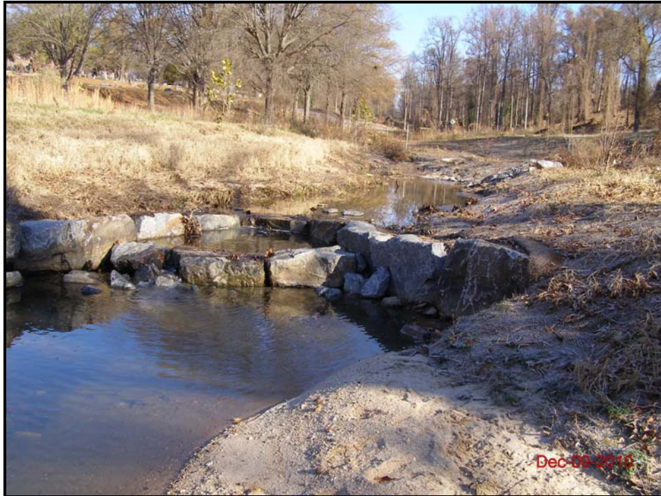
Dye Branch – Permanent Photo Station 4 Looking Upstream
