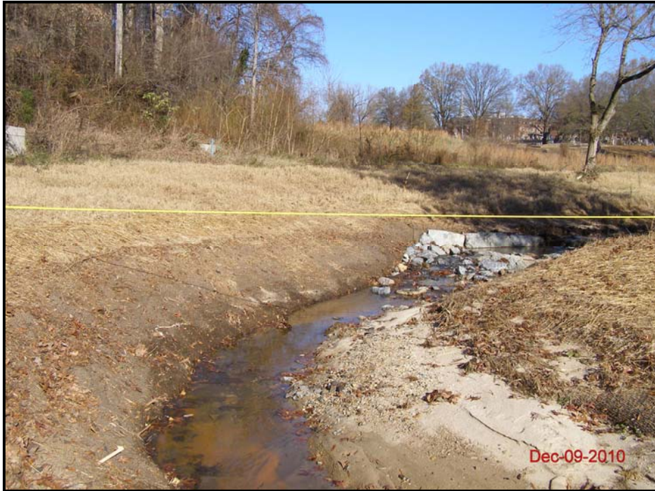
Dye Branch Upstream – Cross-Section 5 – Pool (Looking Upstream) Baseline – December 9, 2010
