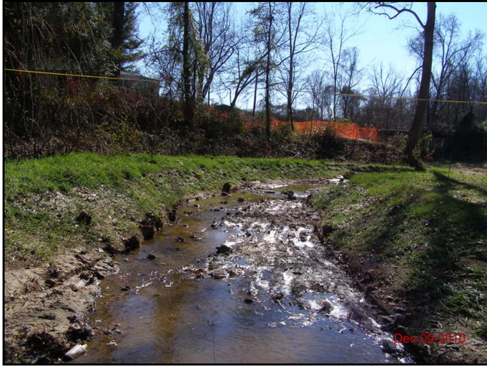
Dye Branch Downstream – Cross-Section 10 – Riffle (Looking Downstream) Baseline – December 9, 2010
