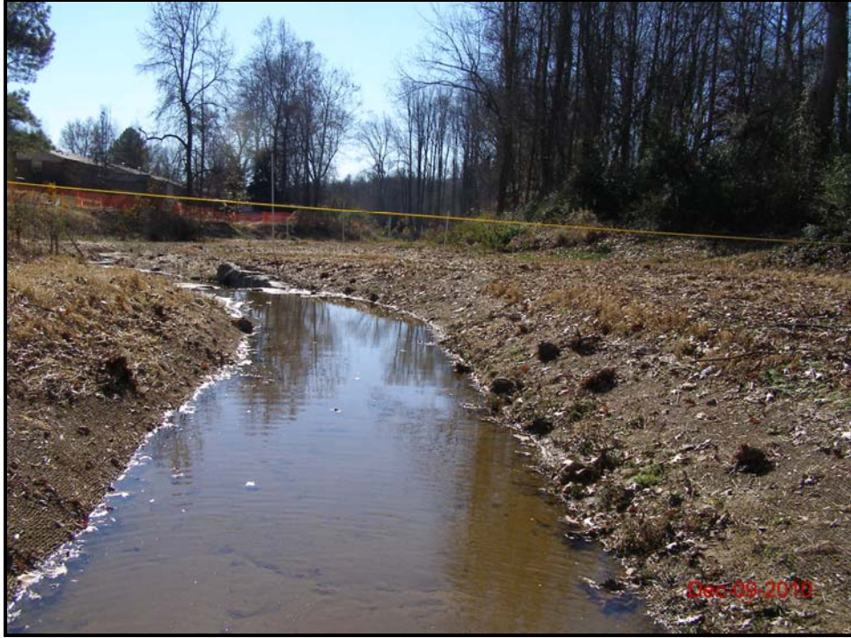
Dye Branch Downstream– Cross-Section 8 – Riffle (Looking Downstream) Baseline – December 9, 2010
