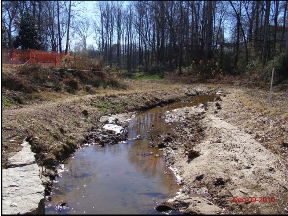
Dye Branch Downstream – Cross-Section 9 – Pool (Looking Downstream) Baseline – December 9, 2010
