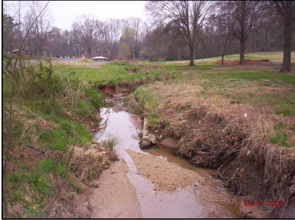
Dye Branch Pre-construction conditions in proximity to Photo Station 3
