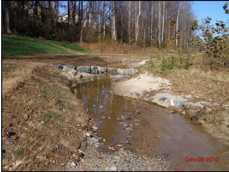
Dye Branch – Permanent Photo Station 9 Looking Upstream
