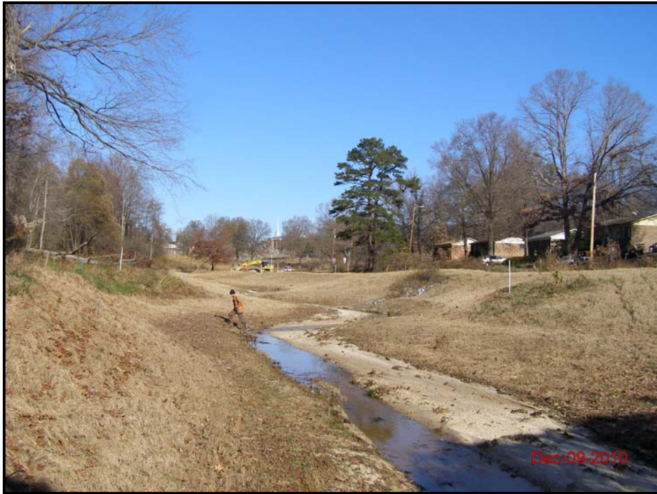
Dye Branch – Permanent Photo Station 6 Looking Upstream
