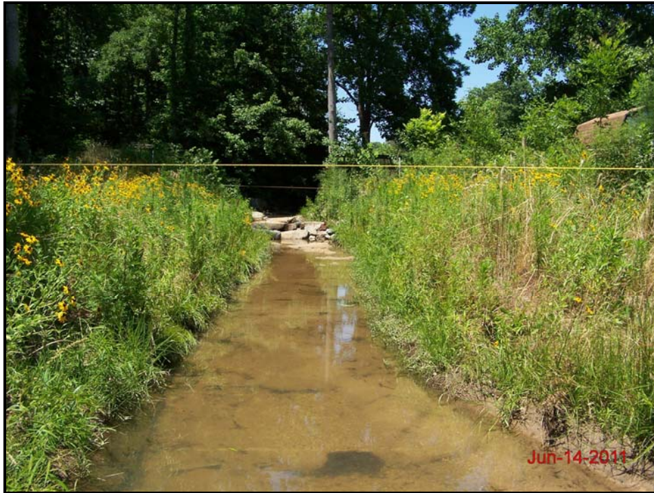
Dye Branch Downstream – Cross-Section 8 – Riffle (Looking Upstream) Monitoring Year 1 – June 14, 2011
