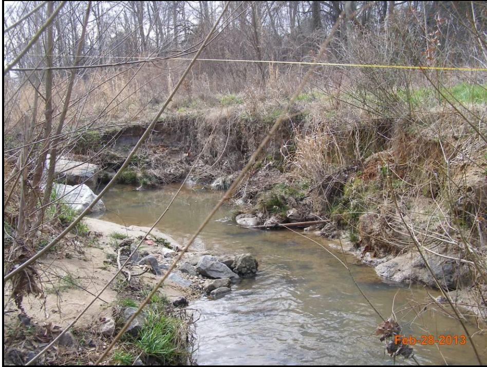
Dye Branch Upstream Reach – Cross-Section 5 – Pool Downstream Monitoring Year 3 – February 28, 2013
