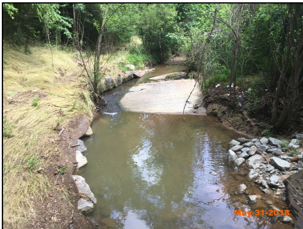
Dye Branch – Permanent Photo Station 11 Downstream Repair Area STA 19+00 (Photo from 2018)
