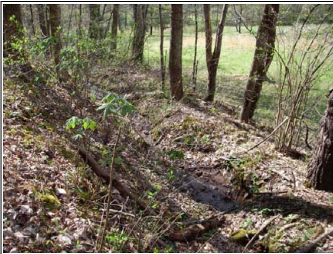
UT2 – Berm along right bank proposed for breaching to re-align channel down valley.
