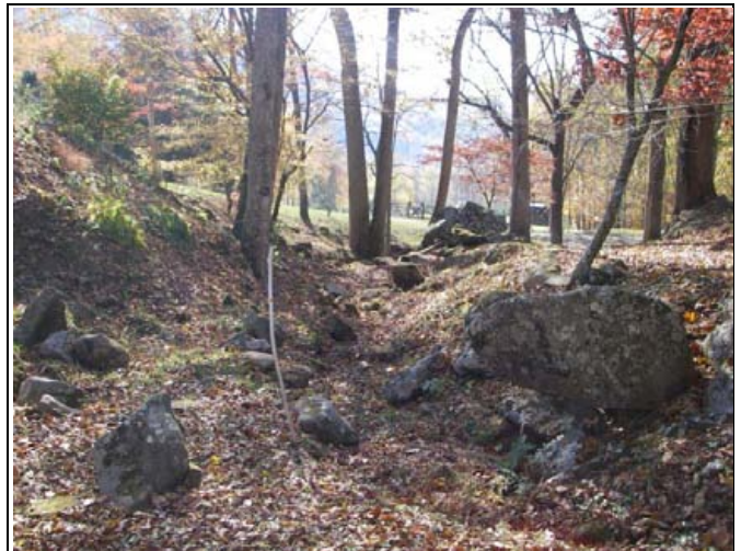
UT2 – ‘Relic’ channel within which UT2 drained before channelization and where flow from the proposed alignment will be re-routed (looking down valley).
