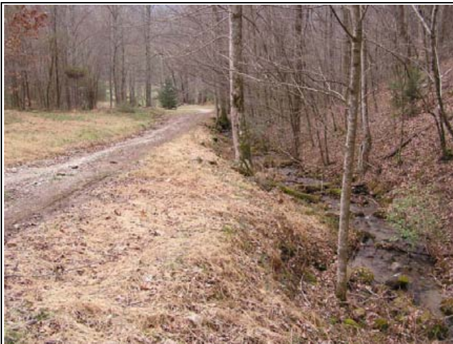
UT6 Reach 3 (enhancement) – Overwidened, entrenched channel with no buffer pinched between valley wall and eroding road embankment.
