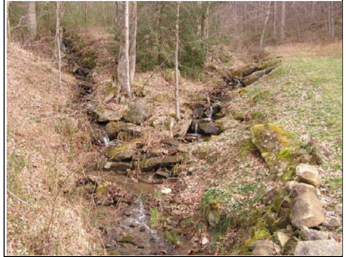
UT5 Reach 2 (enhancement) – Confluence of UT5 Reach 2 and East Buffalo looking upstream.
