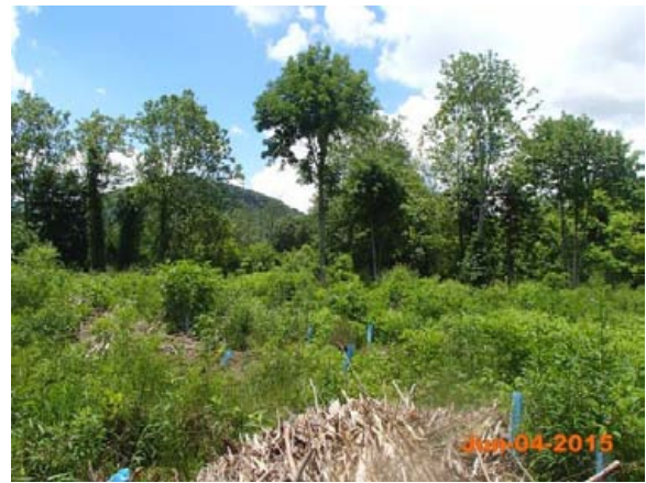
East Fork Pigeon River-Permanent Photo Station 16 West
