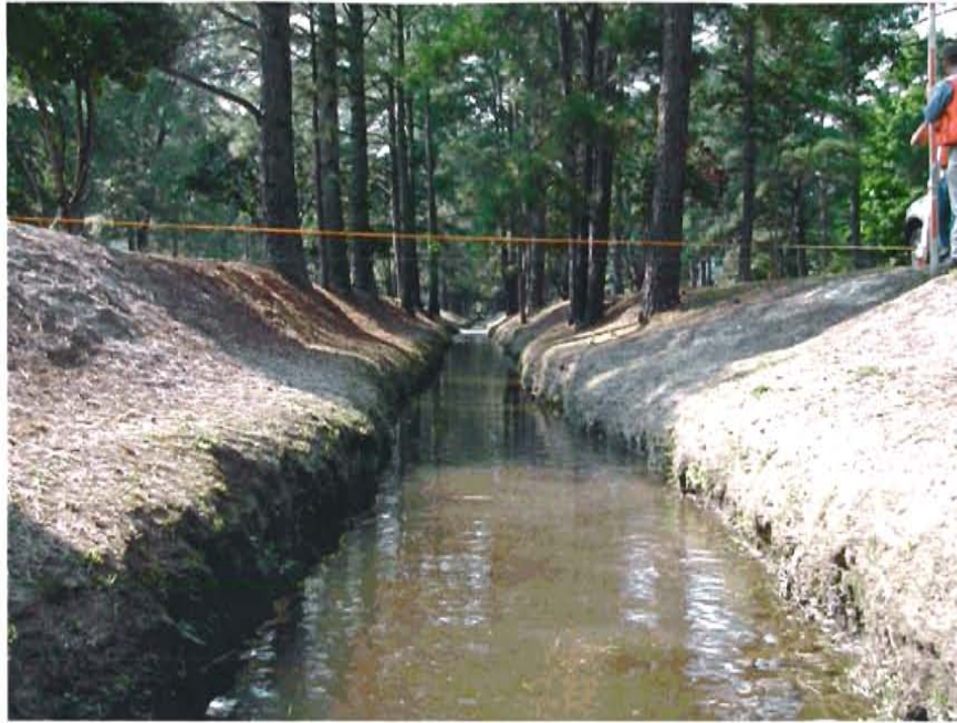
3. Looking downstream from point approximately 150' downstream of Forest Acres Drive culvert
