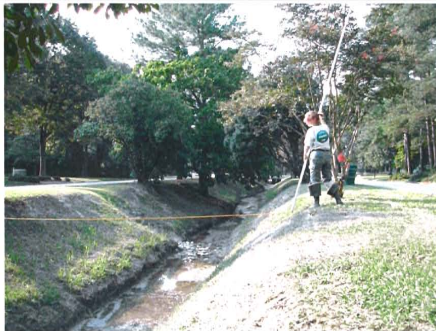
4. Looking downstream from point just downstream of Clark Drive culvert
