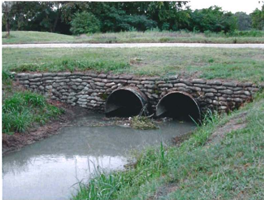
9. Looking downstream at Wilson Street culvert
