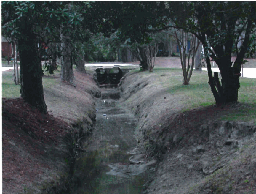
2. Looking upstream at Forest Acres Drive culvert
