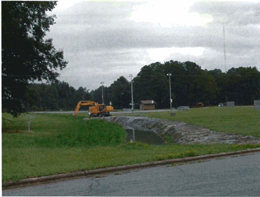
7. Looking upstream from Wilson Street during Town “maintenance” of canal
