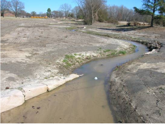
Photo Point 11. Culvert at St. James St. (End of Reach 2). Station 39+88.
