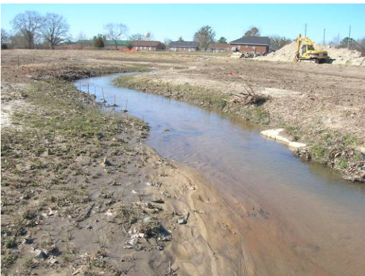
Cross Section 6. Facing downstream. Station 13+97.
