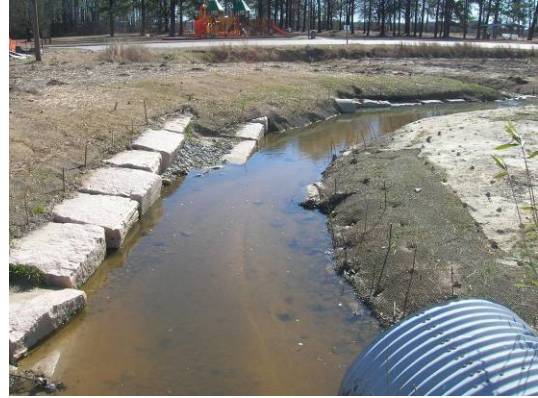
Photo Point 5. Culvert at beginning of Reach 2 facing downstream. Station 10+00.
