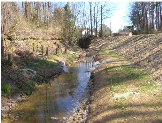
Cross Section 5. Facing downstream. Station 27+29.
