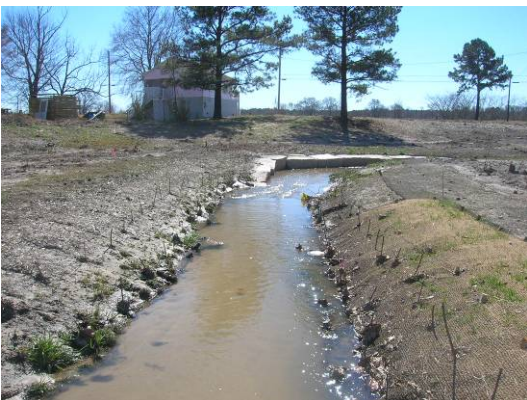
Cross Section 13. Facing downstream. Station 36+91.
