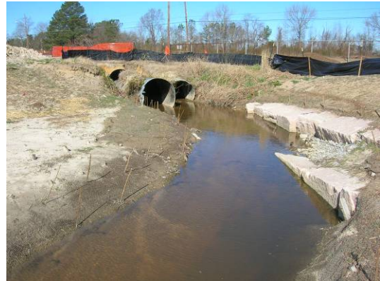
Photo Point 6. At culvert facing upstream. Station 10+57.
