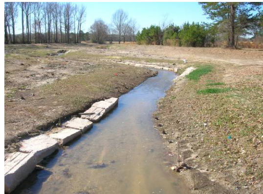
Photo Point 8. Culvert at Wilson St. facing downstream. Station 23+00.
