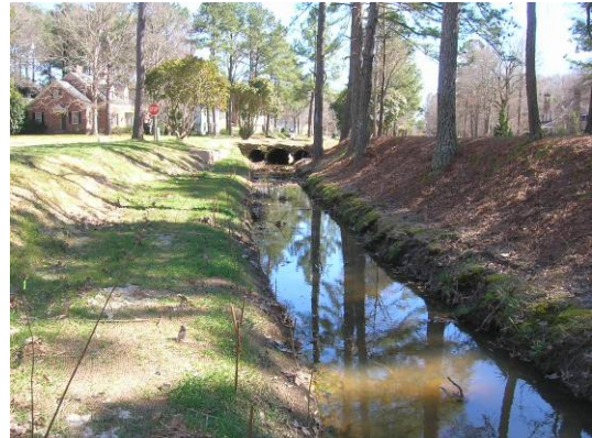
Cross Section 2. Facing downstream. Station 18+08.
