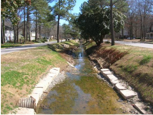
Photo Point 3. Culvert at Clark St. facing downstream. Station 19+82.
