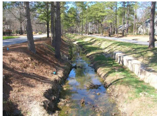
Photo Point 2. Culvert at Clark St. facing upstream. Station 19+47.
