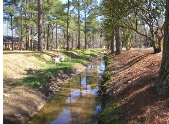
Cross Section 1. Facing downstream. Station 12+71
