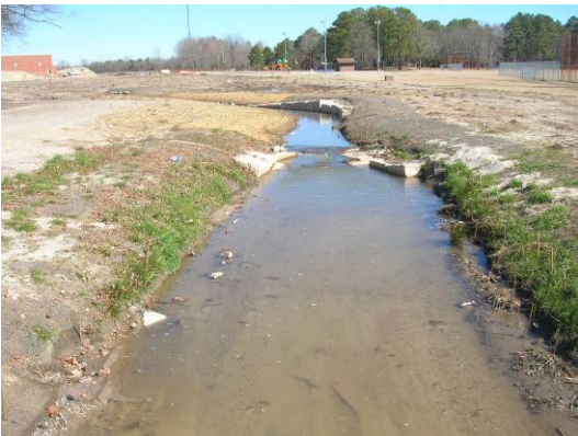
Photo Point 7. Culvert at Wilson St. facing upstream. Station 22+24
