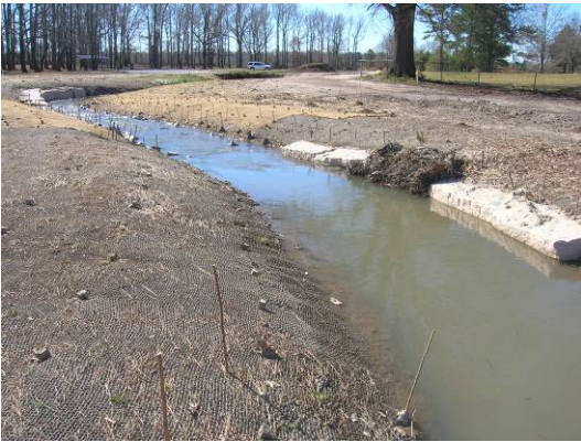
Cross Section 8. Facing downstream. Station 19+93.
