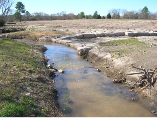
Cross Section 12. Facing downstream. Station 33+80.
