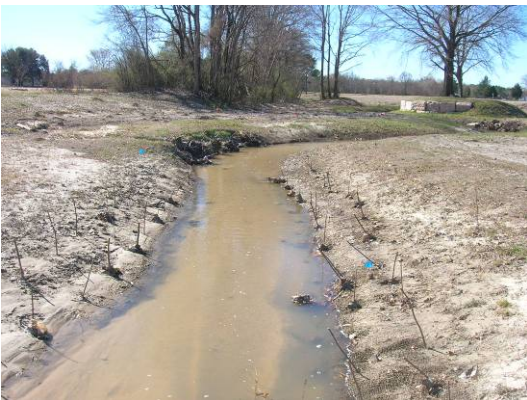
Cross Section 11. Facing downstream. Station 30+15.
