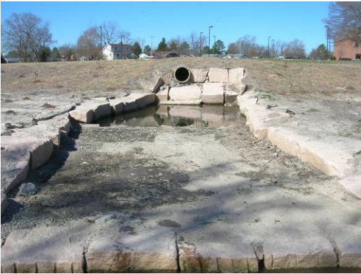
Photo Point 9. Facing Culvert. Station 34+25.
