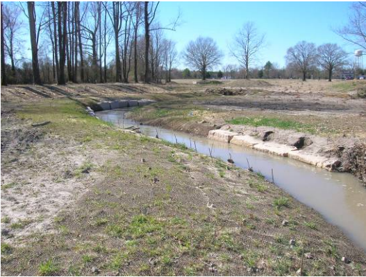
Cross Section 10. Facing downstream. Station 26+76.
