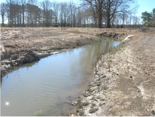
Cross Section 7. Facing downstream. Station 17+86.
