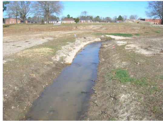
Cross Section 9. Facing downstream. Station 24+78.
