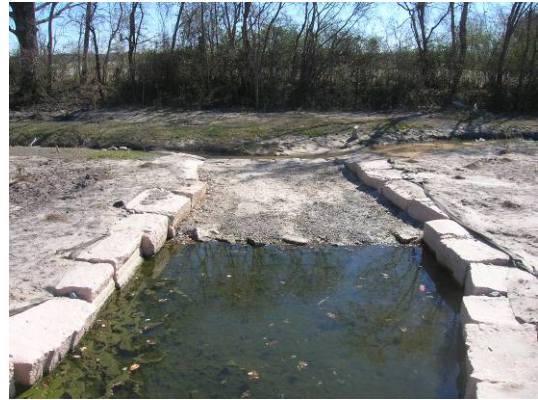
Photo Point 10. On culvert facing stream. Station 34+13 offset 58.05.
