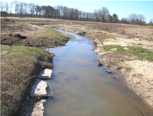
Photo Point 6. At culvert facing downstream. Station 10+57.
