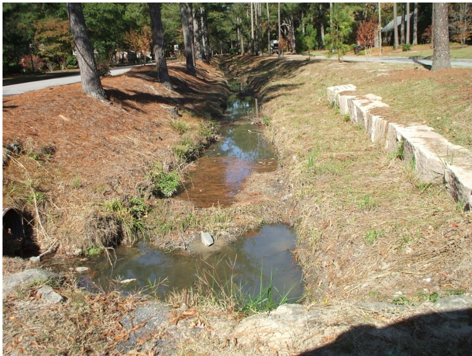
Photo Station 2. Reach 1 Culvert upstream
