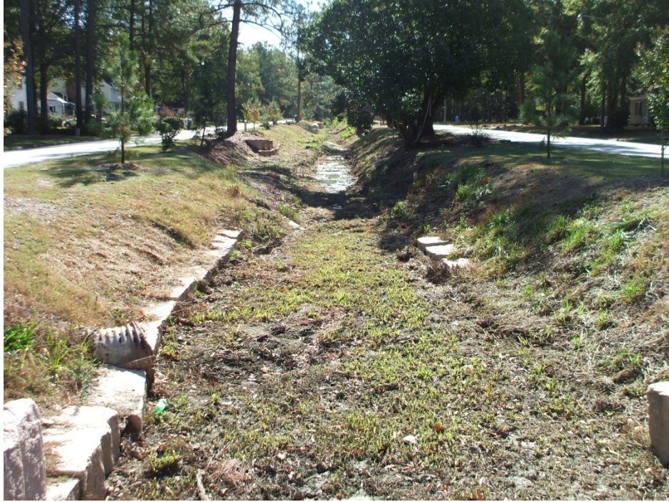
Photo Station 3. Reach 1 Culvert Downstream
