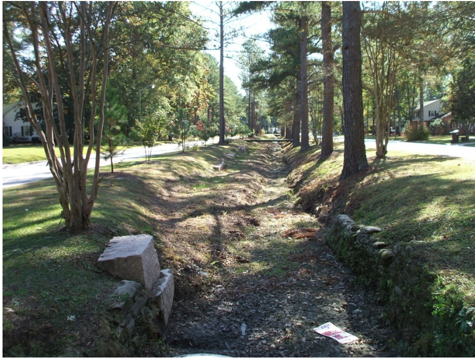
Photo Station 1. Beginning of Reach 1
