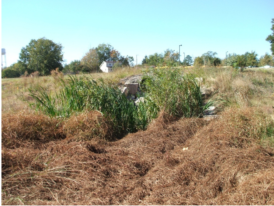
Photo Station 9. Culvert Upstream
