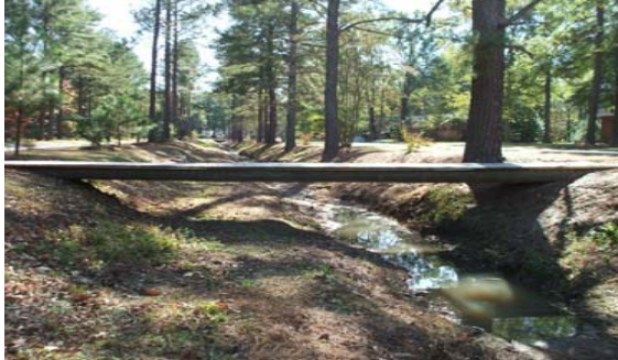
Photo of Cross-Section #1 - Looking Downstream
