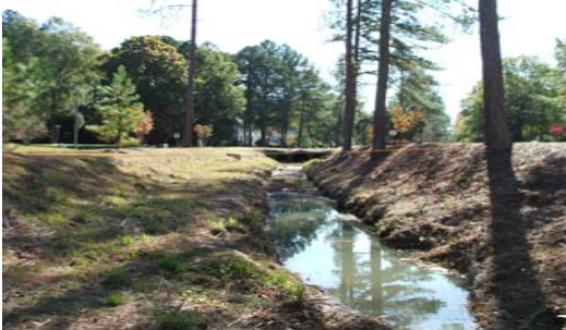
Photo of Cross-Section #2 - Looking Downstream
