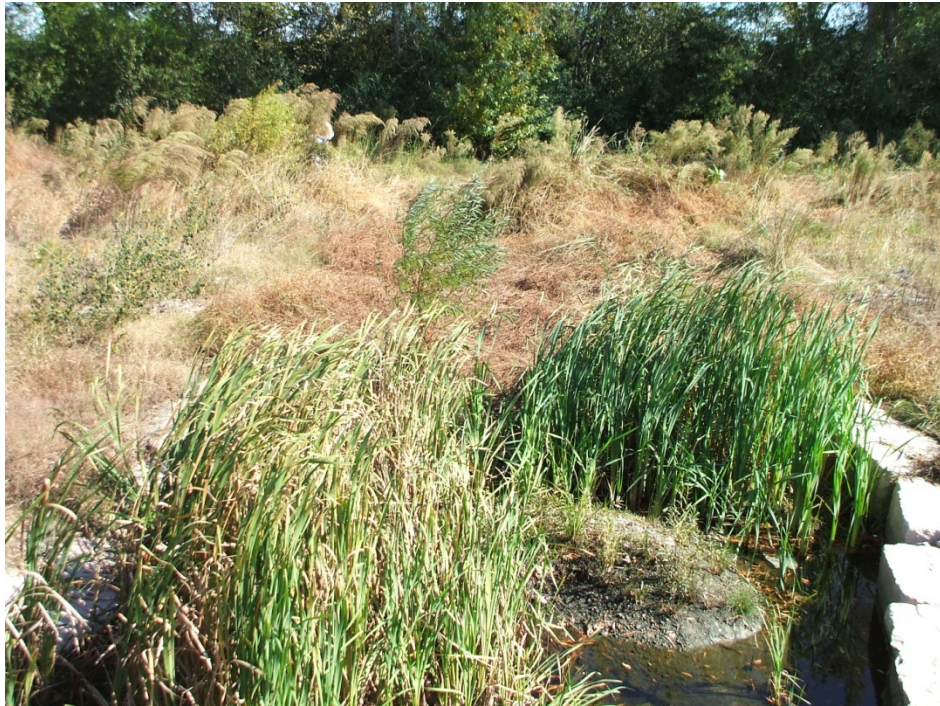
Photo Station 10. Pool Culvert Downstream
