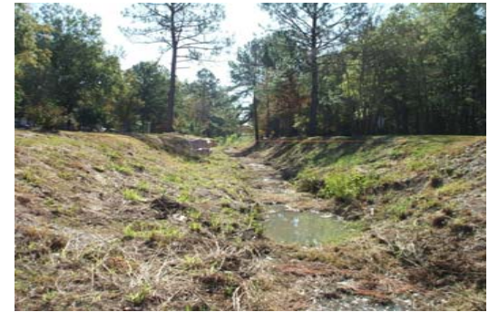
Photo of Cross-Section #4 - Looking Downstream
