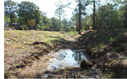
Photo of Cross-Section #3 - Looking Downstream
