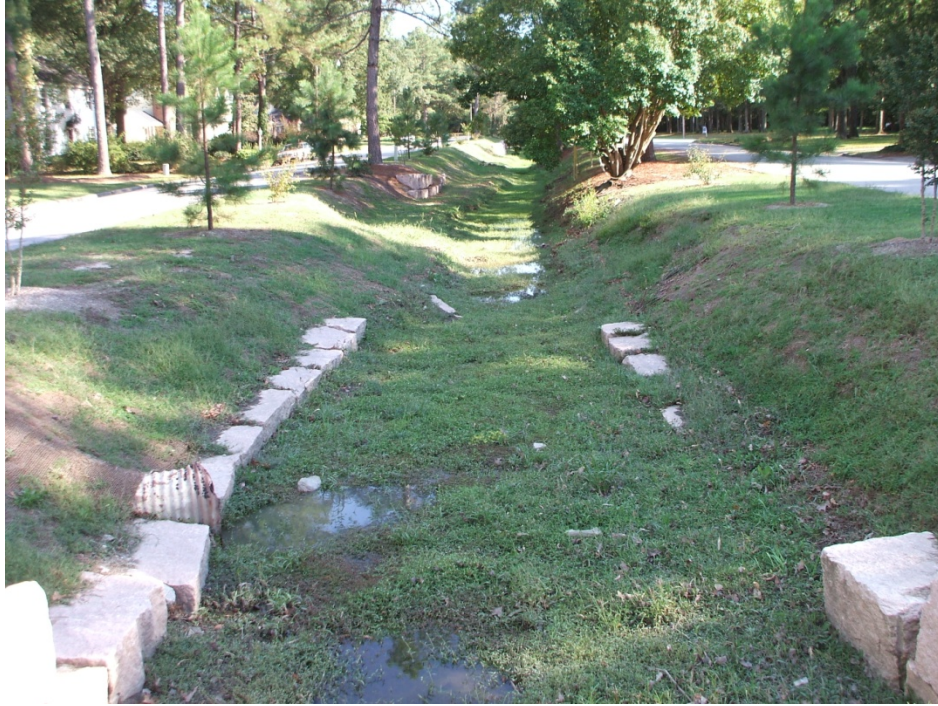
Photo Station 3. Reach 1 Culvert Downstream
