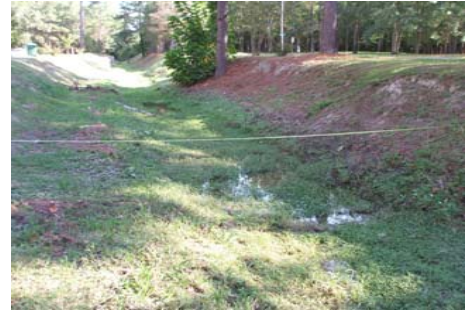
Photo of Cross-Section #3 - Looking Downstream
