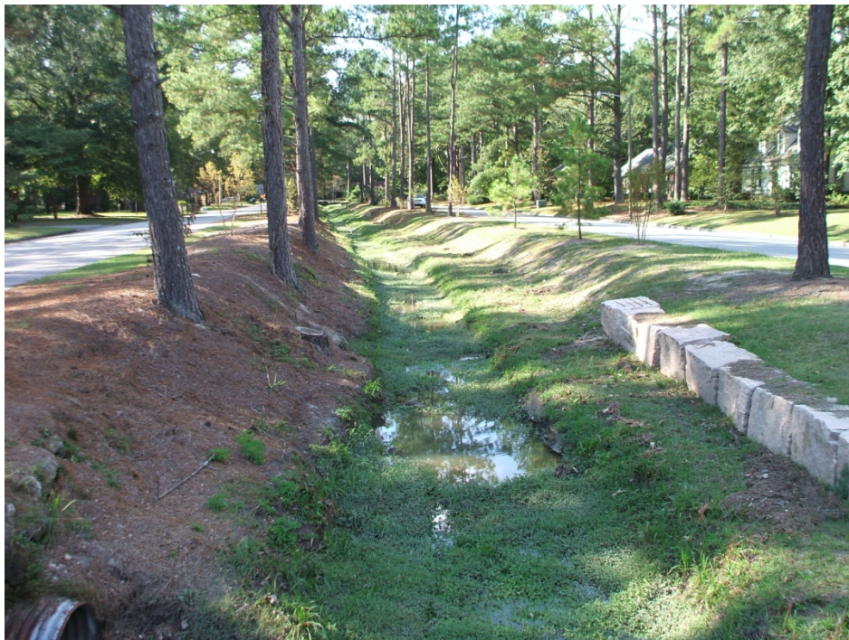
Photo Station 2. Reach 1 Culvert upstream
