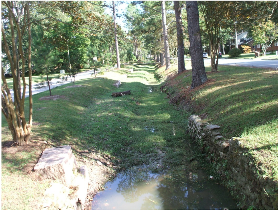
Photo Station 1. Beginning of Reach 1
