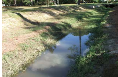
Photo of Cross-Section #2 - Looking Downstream
