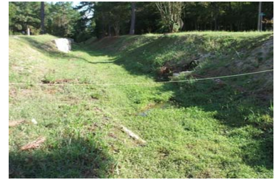
Photo of Cross-Section #4 - Looking Downstream
