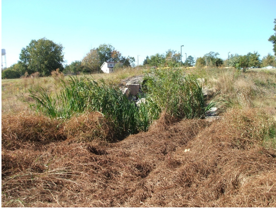
Photo Station 9. Culvert Upstream
