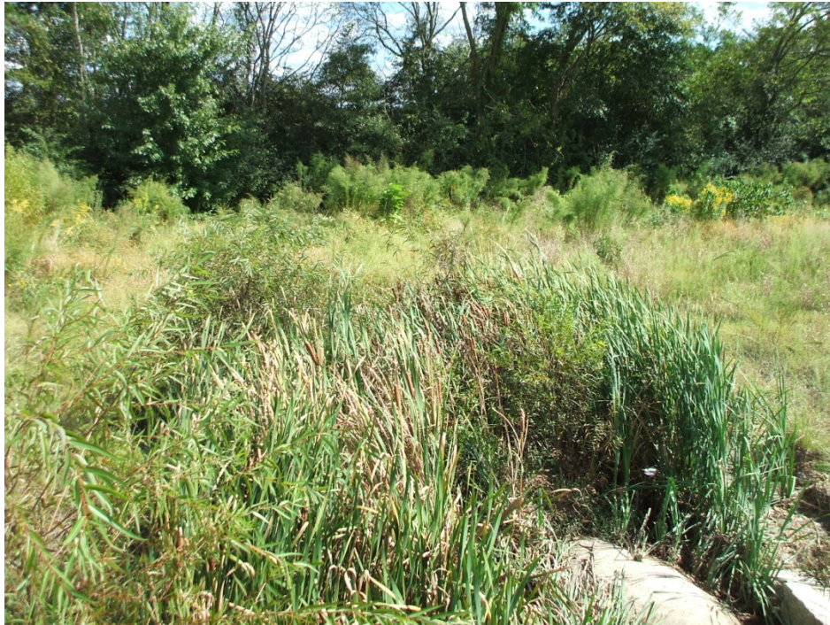
Photo Station 10. Pool Culvert Downstream
