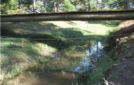
Photo of Cross-Section #1 - Looking Downstream
