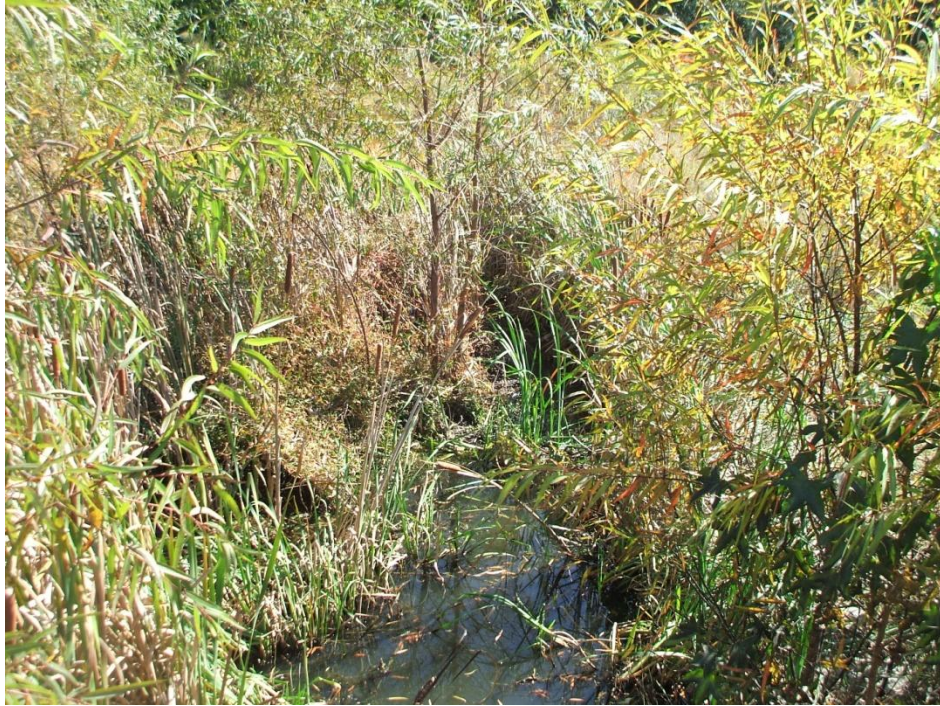
Photo Station 9. Culvert Upstream
