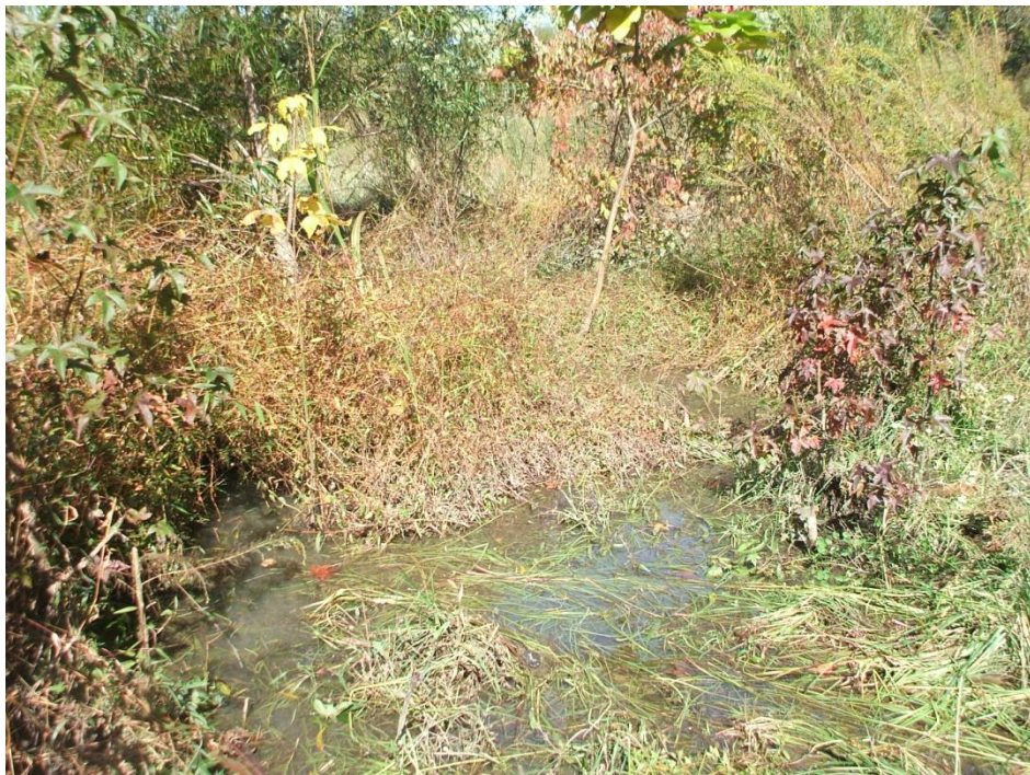
Photo Station 10. Pool Culvert Downstream
