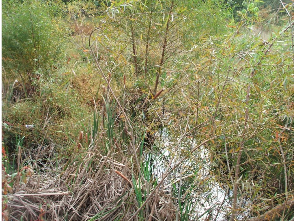
Photo Station 9. Culvert entry downstream
