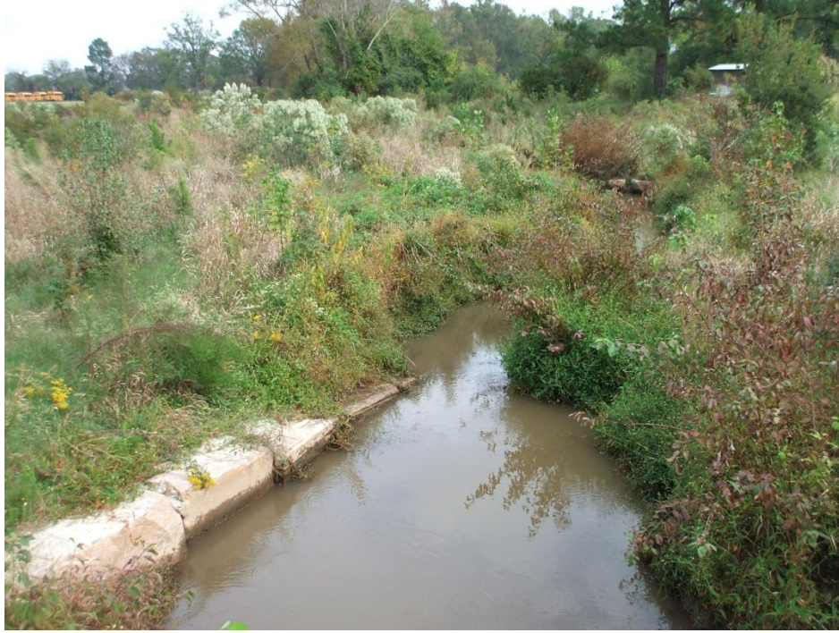
Photo Station 11. Reach 2 End of Project
