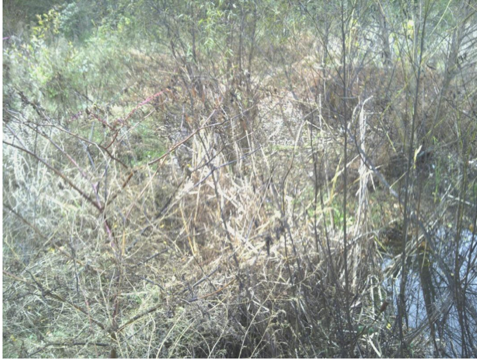
Photo Station 9. Culvert entry downstream
