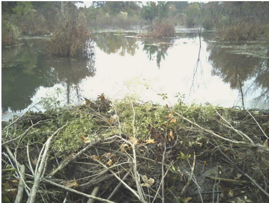
SP2 – Beaver Dam and ponding - Sta. 29+50 - Reach 2
