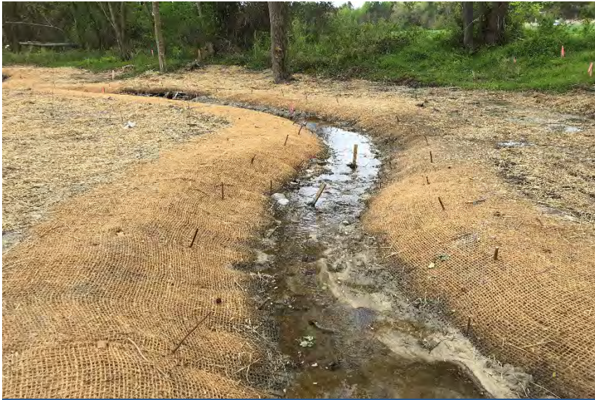
PS-5, Reach R2, facing downstream, Sta 19+50, Sept 17, 2018 (MY-00)
