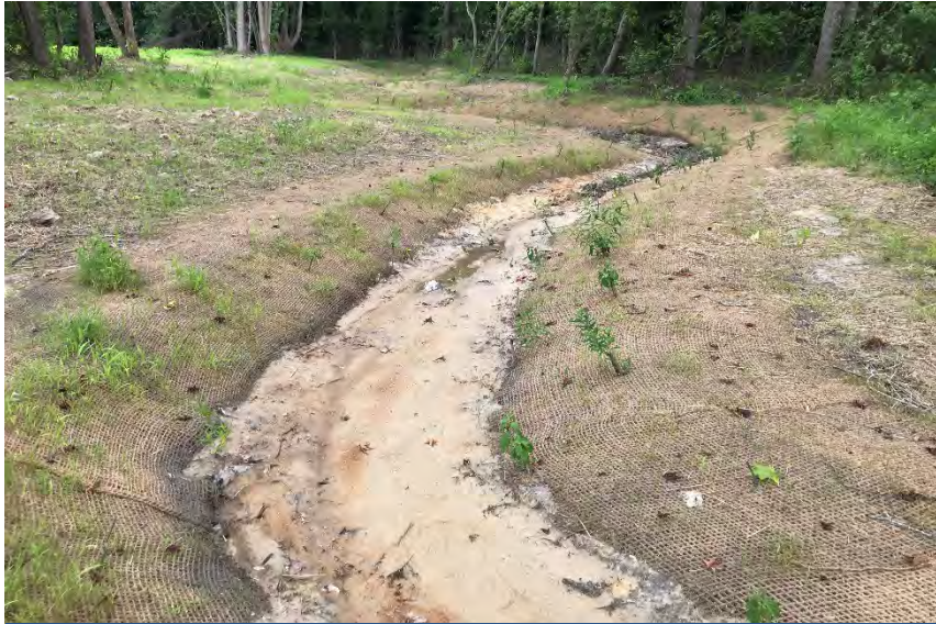
PS-11, Reach R4, facing upstream, Sta 13+00, June 11, 2018 (MY-00)
