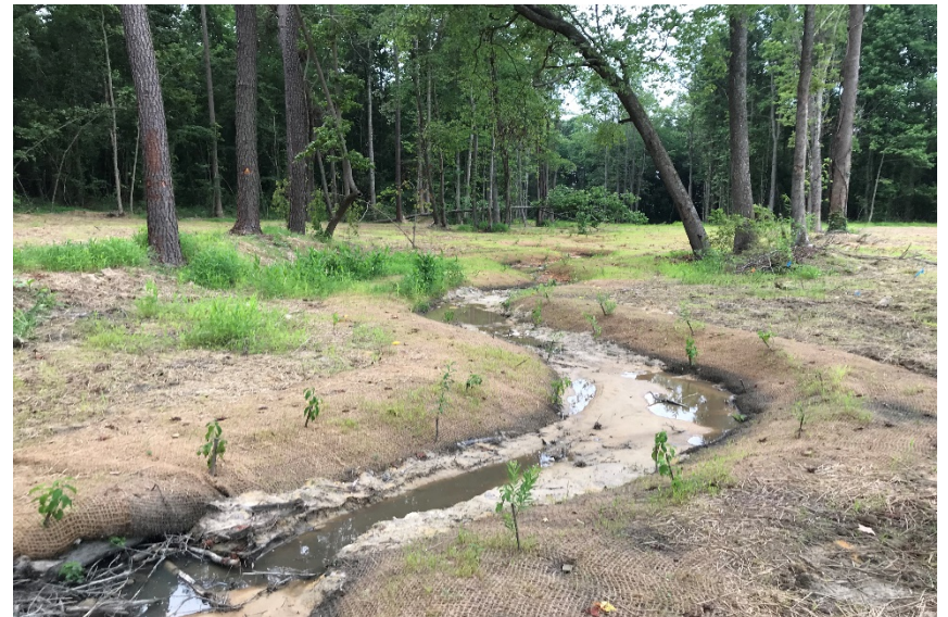
Reach R4, facing downstream, Sta 13+00, June 11, 2018 (MY-00)
