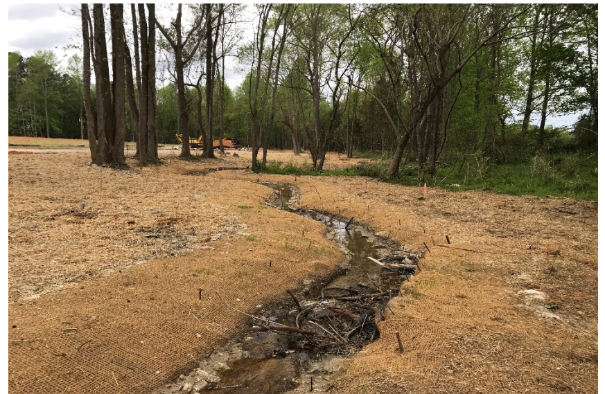
Reach R2, facing downstream, Sta 18+00, April 23, 2018 (MY-00)
