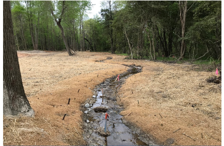
Reach R2, facing downstream, Sta 21+00, April 23, 2018 (MY-00)
