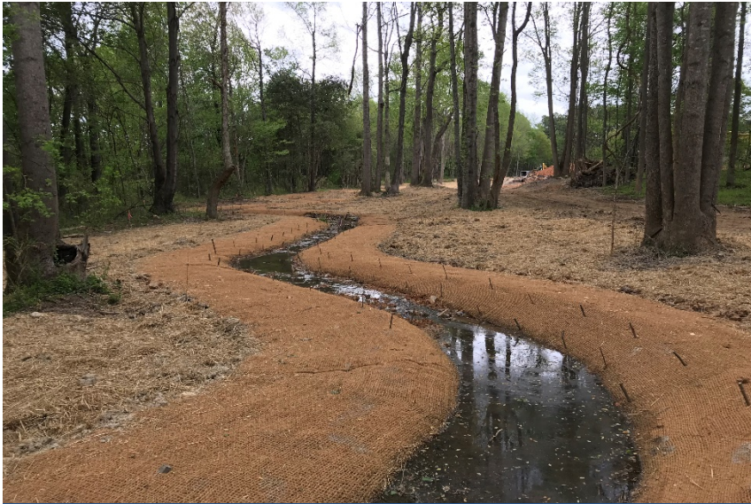
Reach R2, facing upstream, Sta 26+00, April 23, 2018 (MY-00)
