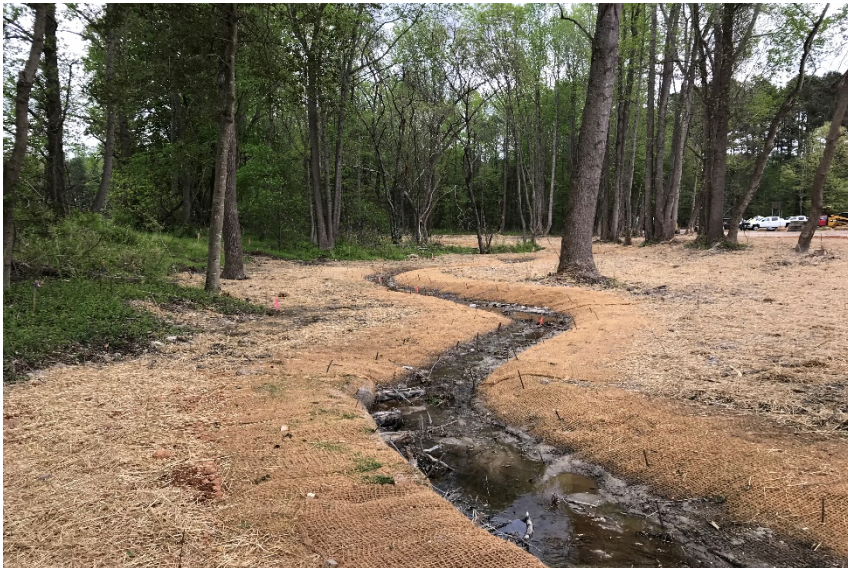
Reach R2, facing upstream, Sta 21+00, April 23, 2018 (MY-00)
