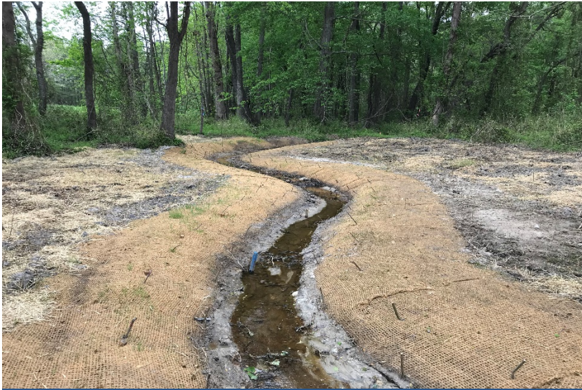
Reach R2, facing upstream, Sta 17+00, April 23, 2018 (MY-00)
