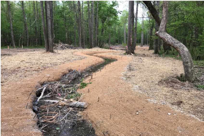
Reach R2, facing downstream, Sta 25+00, April 23, 2018 (MY-00)
