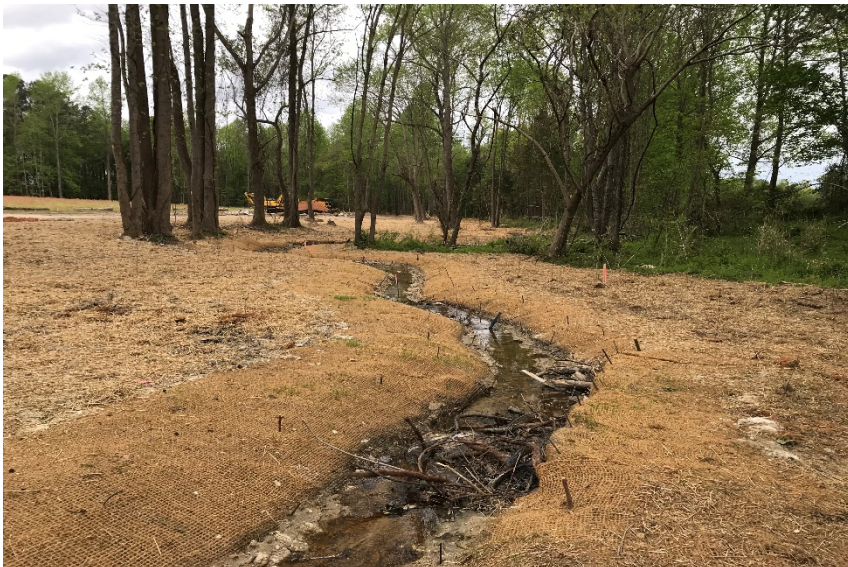
Reach R2, facing downstream, Sta 18+00, April 23, 2018 (MY-00)
