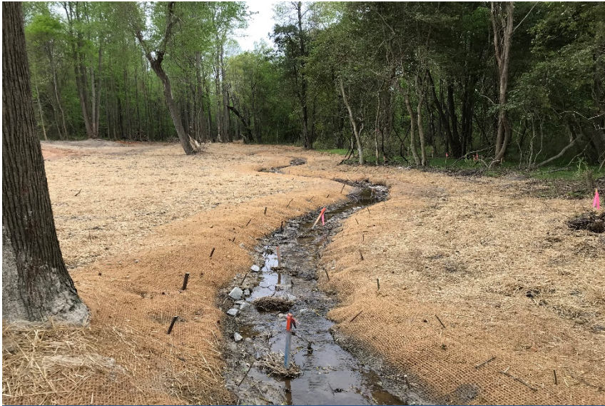
Reach R2, facing downstream, Sta 21+00, April 23, 2018 (MY-00)
