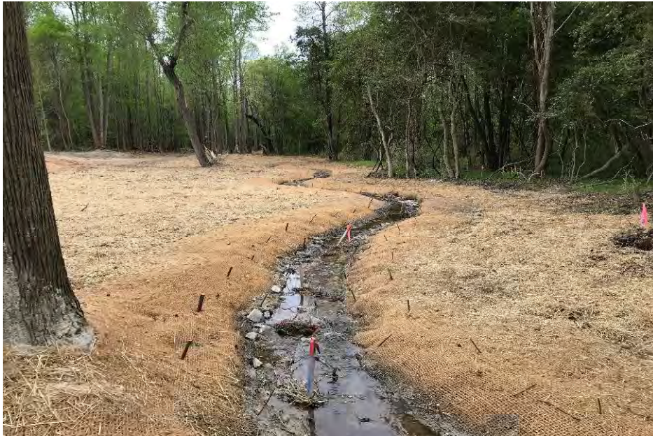
Reach R2, facing downstream, Sta 21+00, April 23, 2018 (MY-00)
