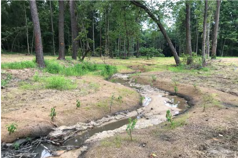
Reach R4, facing downstream, Sta 13+00, June 11, 2018 (MY-00)
