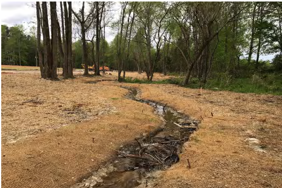
Reach R2, facing downstream, Sta 18+00, April 23, 2018 (MY-00)
