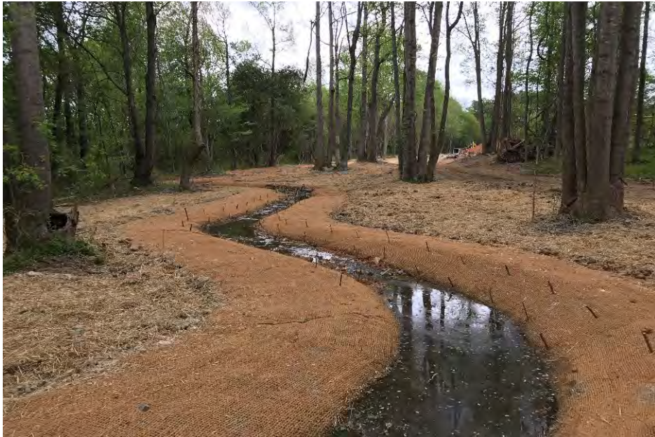
PS-9, Reach R2, facing upstream, Sta 25+75, April 23, 2018 (MY-00)
