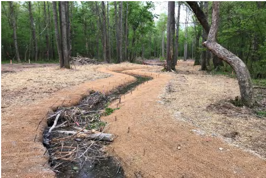
PS-8, Reach R2, facing downstream, Sta 24+50, April 23, 2018 (MY-00)
