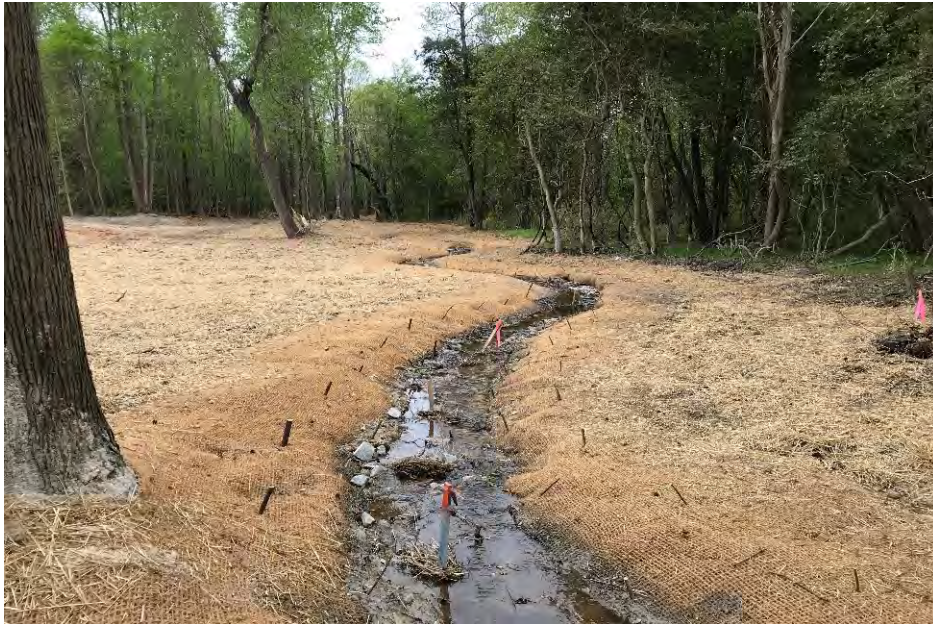
PS-7, Reach R2, facing downstream, Sta 21+00, April 23, 2018 (MY-00)
