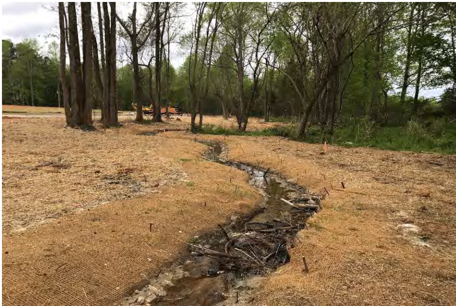
PS-4, Reach R2, facing downstream, Sta 18+00, April 23, 2018 (MY-00)
