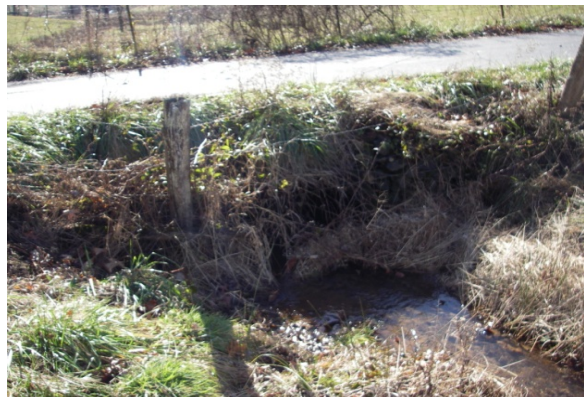
Downstream end of project on Elk Branch Reach 2
