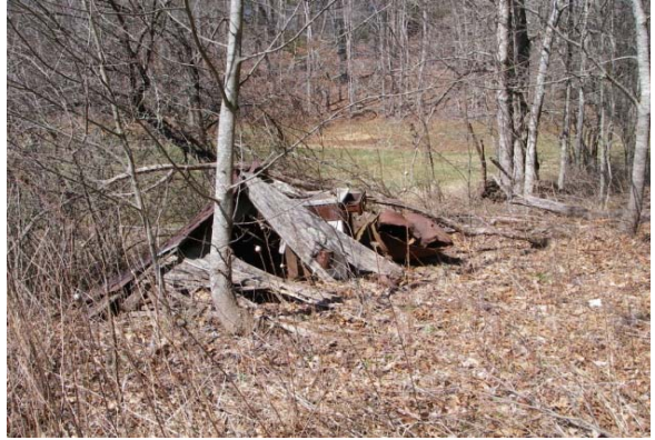
Close-up of UT2 at location of arrow in adjacent photograph (creek buried)
