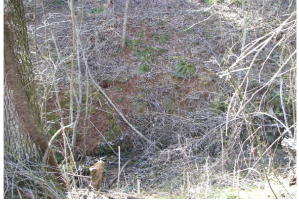
Elk Branch Reach 1 close-up of stream against valley wall and resulting erosion of banks
