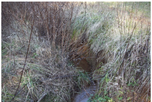
Elk Branch Reach 1 section through field with bank erosion, head cutting, and lack of deep-rooted vegetation
