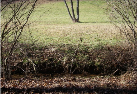
Eroding toe in Elk Branch Reach 2
