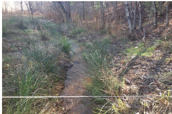
Photo 8: XS-2 facing downstream
