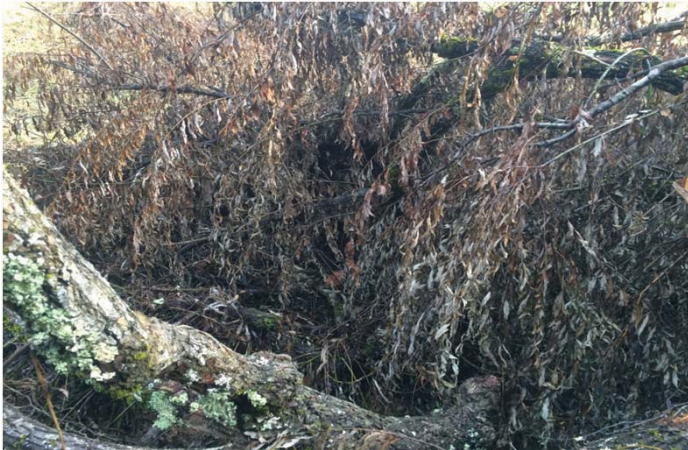
Photo 1: XS-1 facing left bank, showing fallen willow tree laying across transect, storm damage.
