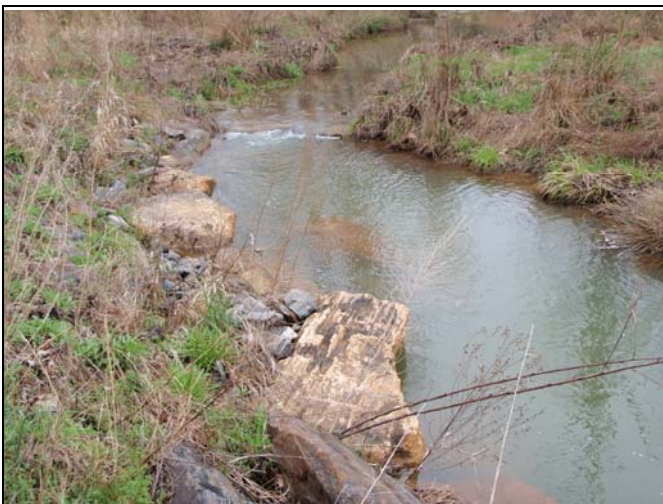
Constructed Riffle 5
