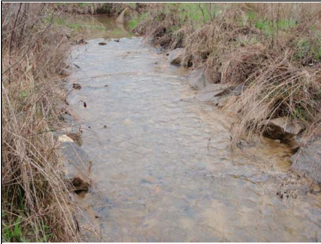
Constructed Riffle 7
