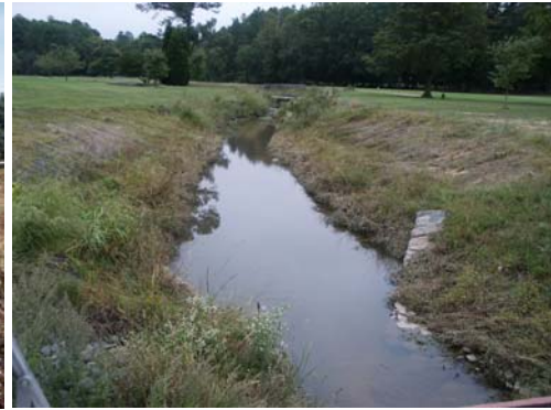
AL-P05 STA 59+21 (BRIDGE)
