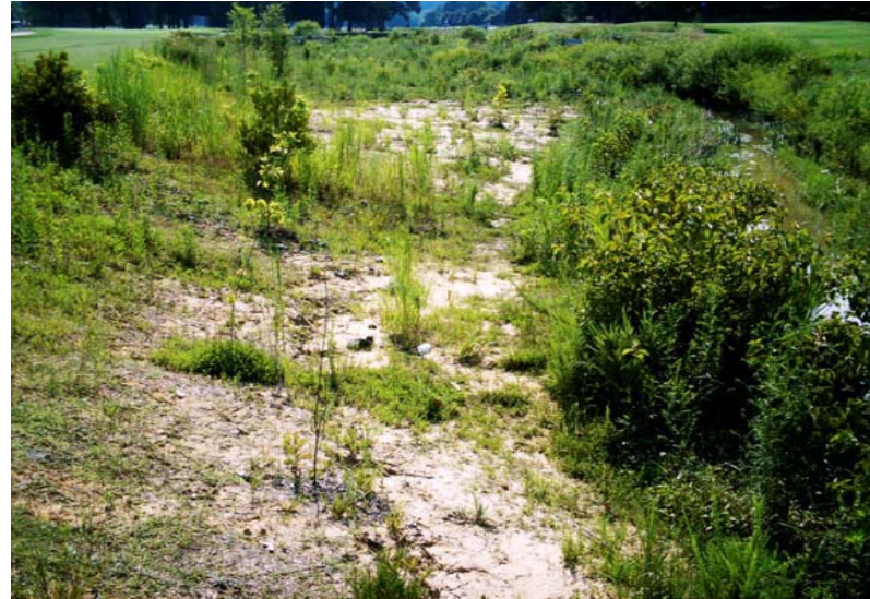
VP2. Bare / eroded soil
