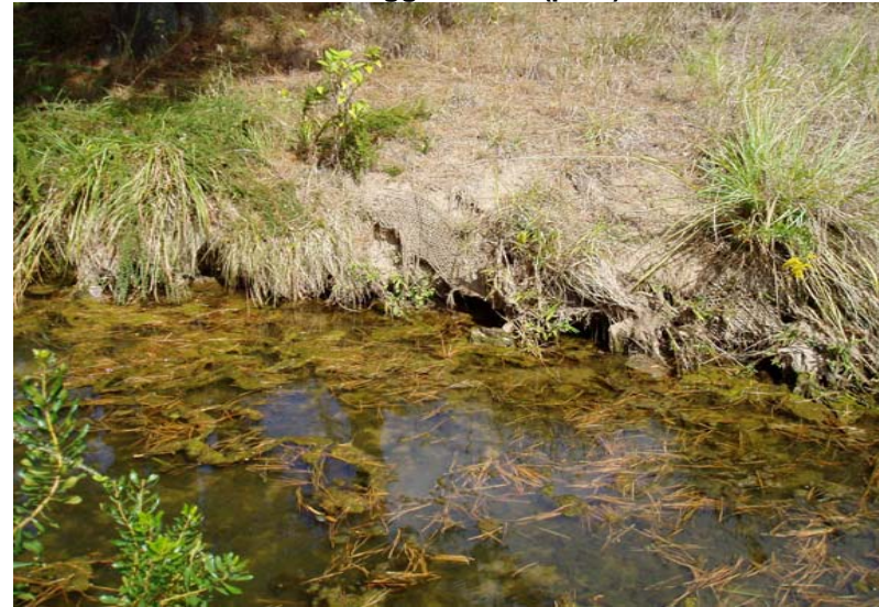
SP4. Bank undercut/scour
