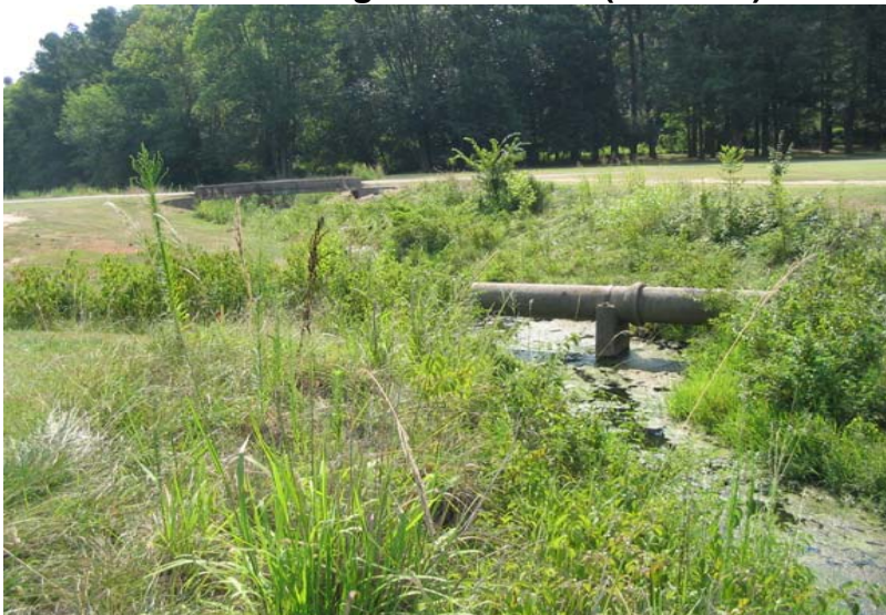
AL-P06 facing downstream (07/27/07)
