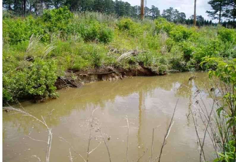
SP6. Bank slump/scour (9/18/08)
