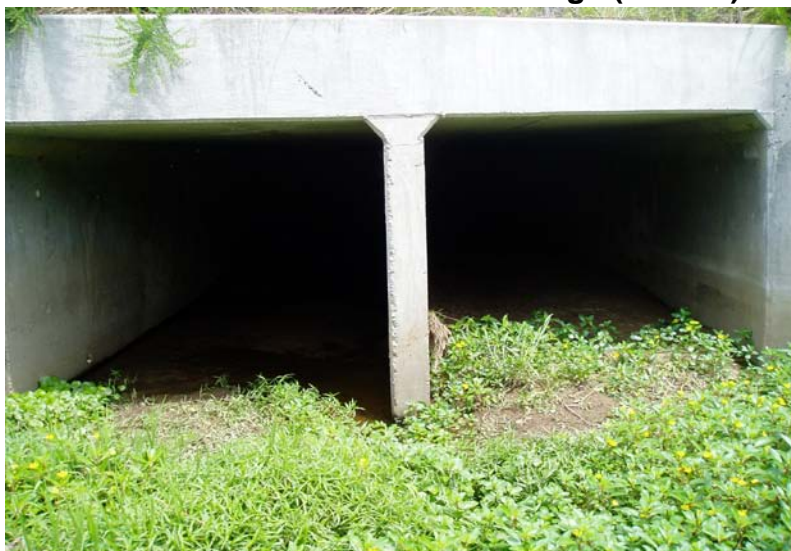
SP11. Aggregation at culvert (9/18/08)
