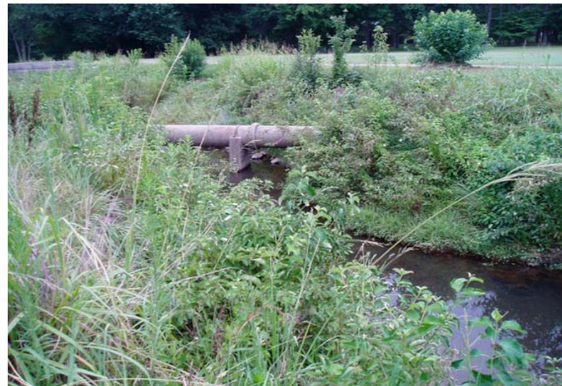
AL-P06 facing downstream (07/25/08)
