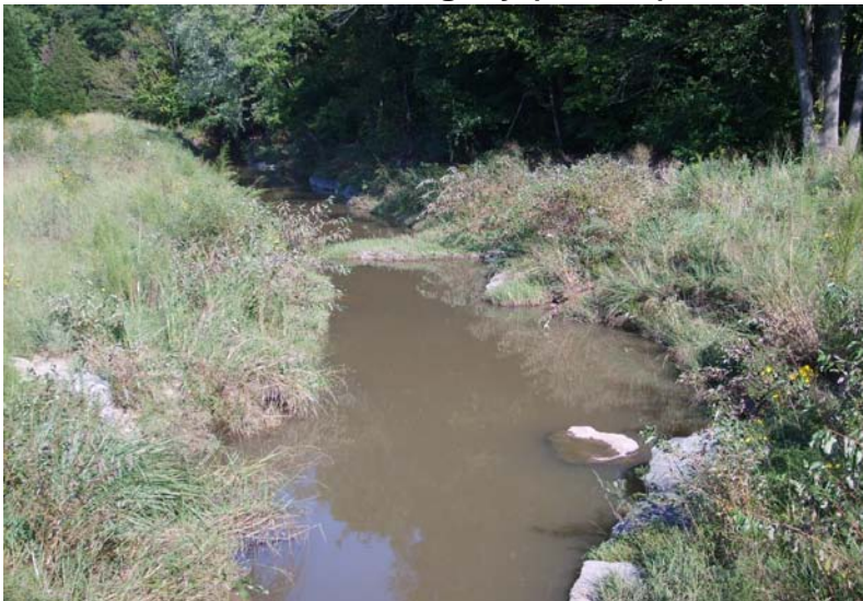
SP7. Boulder failure, banks scour, bar (9/18/08)
