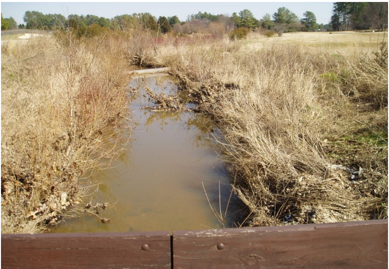
HB-P04 facing downstream (03/06/09)
