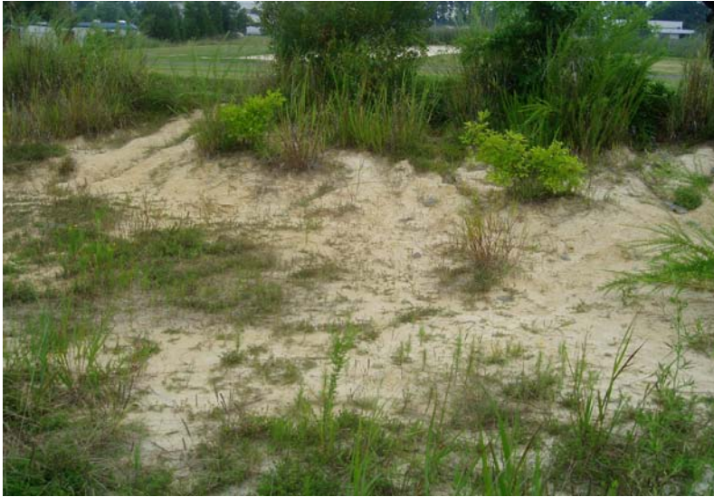
VP1. Bare soil/eroded slopes (7/16/09)
