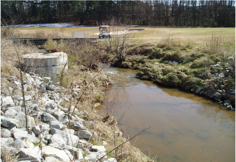
HB-P01 facing downstream (03/06/09)
