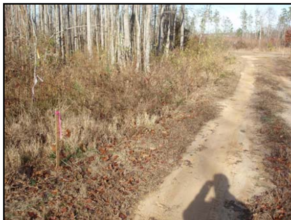
Tributary 4– Tributary flows through culvert under road crossing
