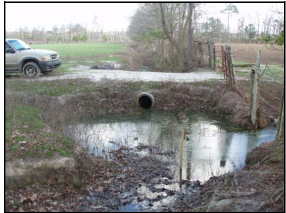
Tributary 2A– Culvert
