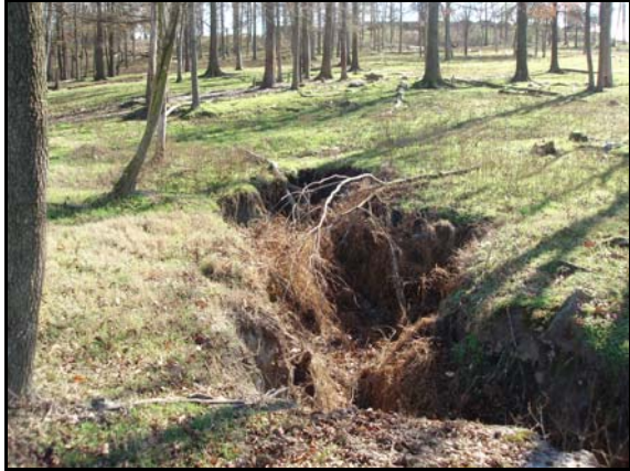
Tributary 1.1– Headcut 2 further downstream
