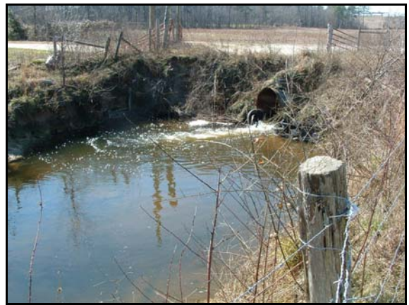
NPAC- View of culvert crossing
