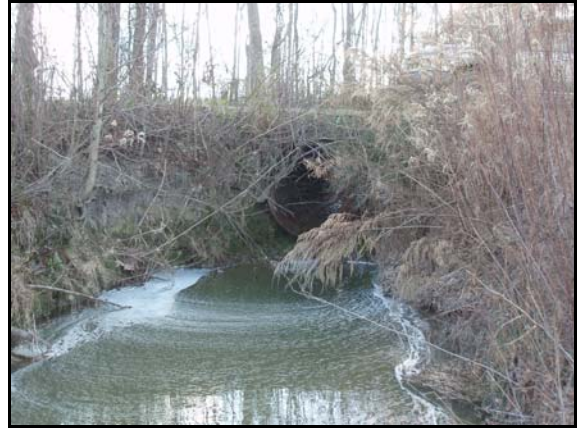
Tributary 3- Tributary at culvert
