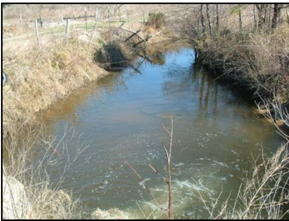
NPAC- View of stream at culvert crossing
