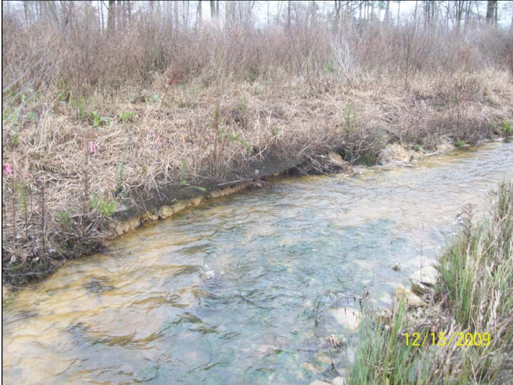
Erosion along toe of bank under coir matting near Station 55+25. MY01 – 12/15/09
