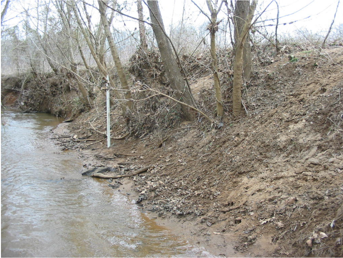
Photo 7: Stable bank on Fifth Creek
