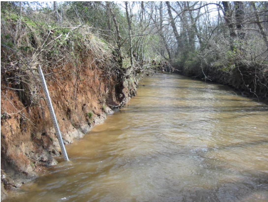
Photo 10: Typical eroding bank on Fifth Creek and moderate right bank
