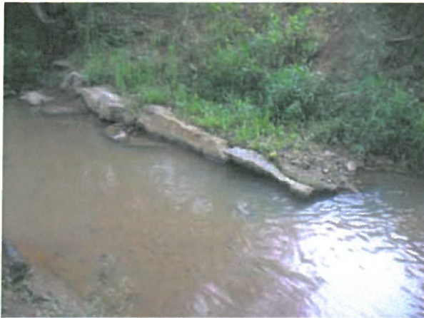
Photo Point 1. Boulder Vane 7/10/12
