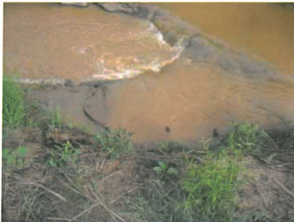
Photo Point 25. Cross Vane. Left arm scour. 7/10/12
