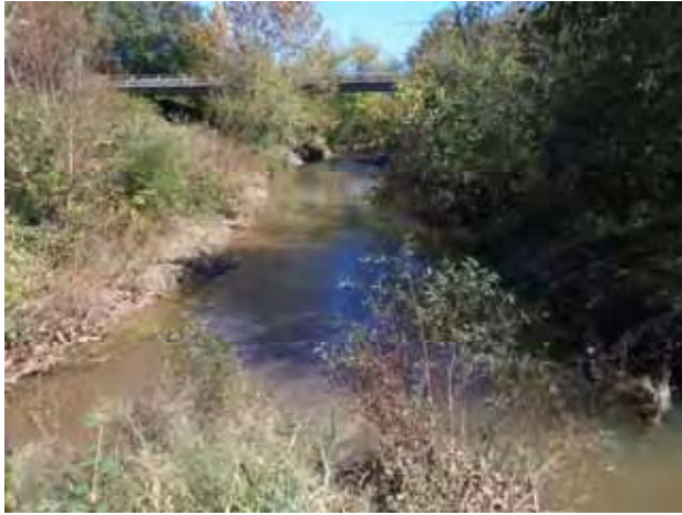
Photo Point 28. Confluence looking east 10/17/14
