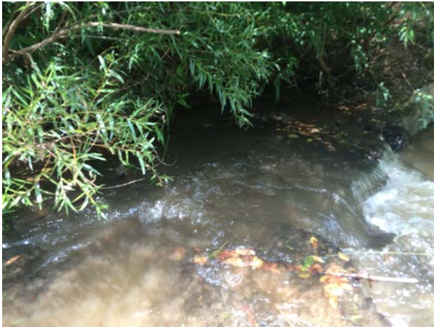
Photo Point 25. Cross Vane. Left arm scour. 08/13/15
