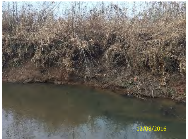
Bank Erosion 67+00 FTH
