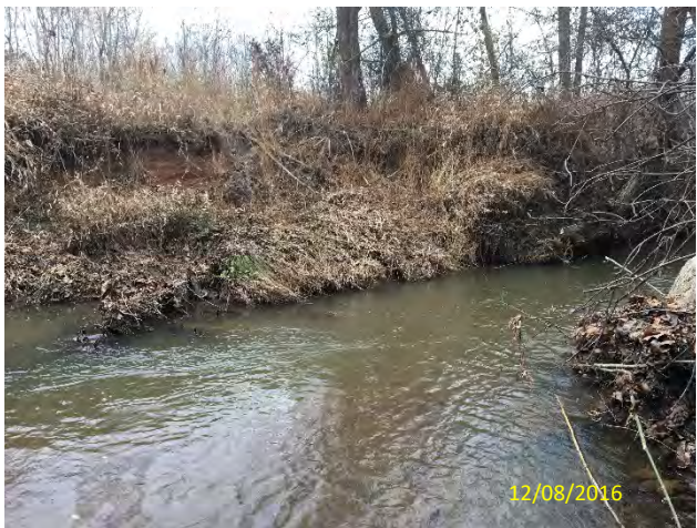
Bank Erosion 54+00 FTH
