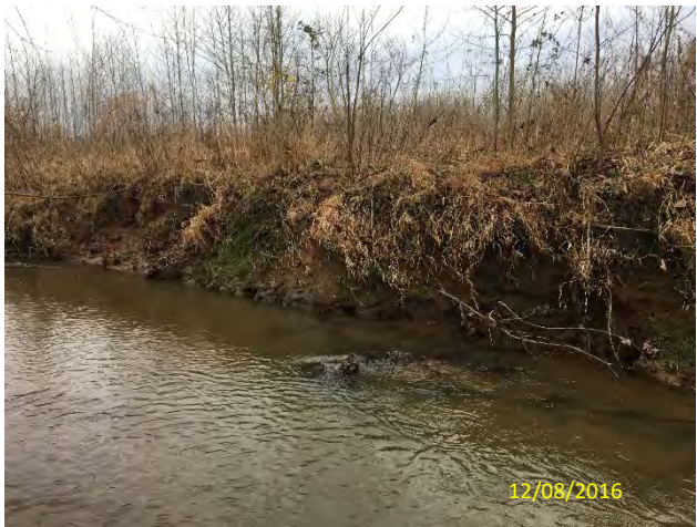
Bank Erosion 52+00 FTH
