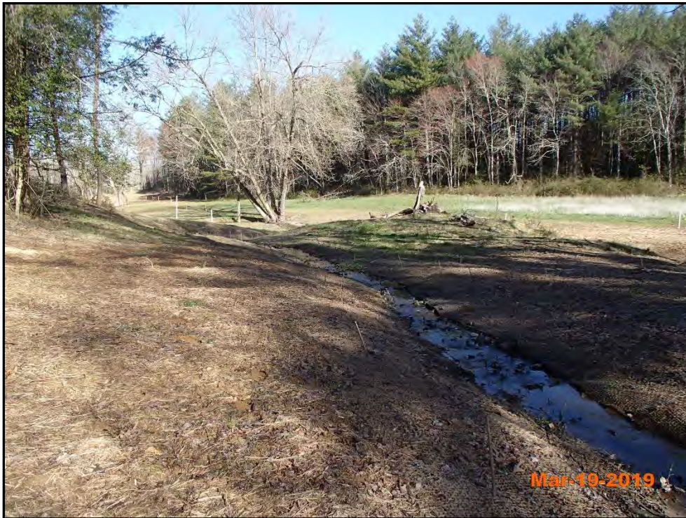
Raccoon Branch 1D – Permanent Photo Station 27 Looking Downstream
