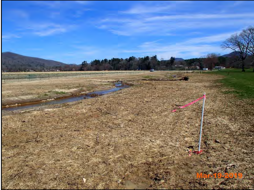
Fletcher Creek 2B – Permanent Photo Station 15 Looking Upstream
