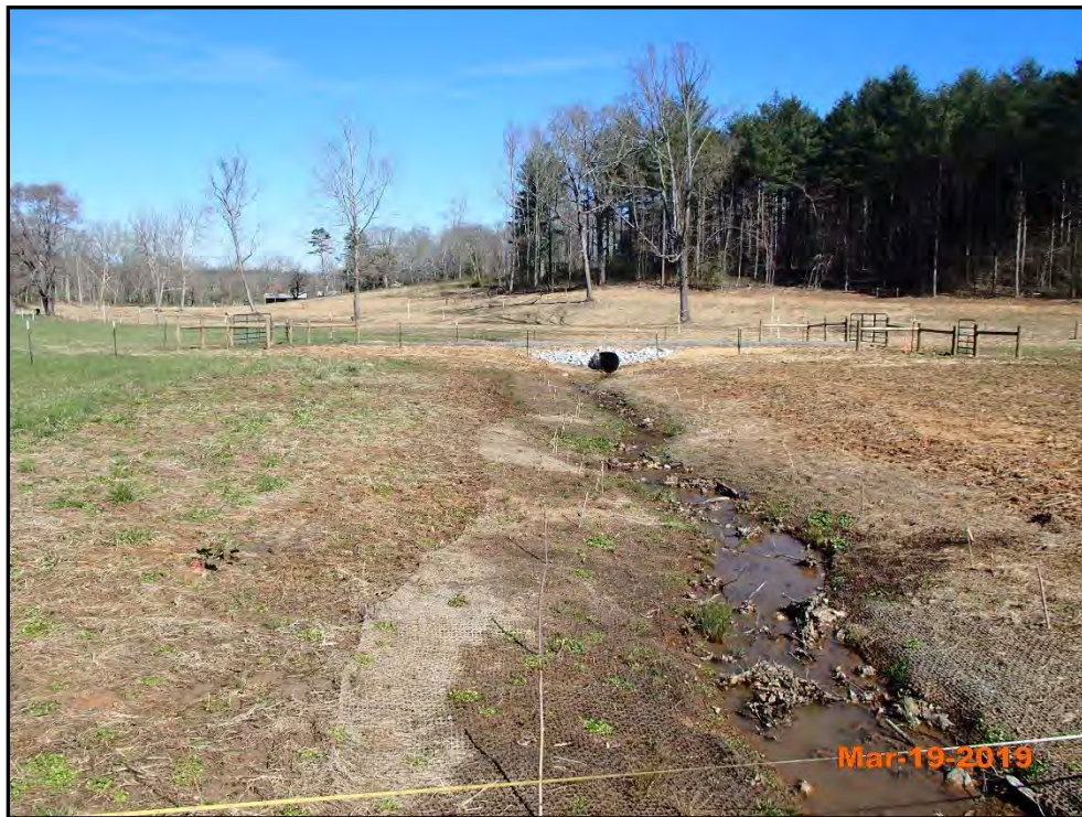
Coats Branch 1B – Permanent Photo Station 30 Looking Downstream
