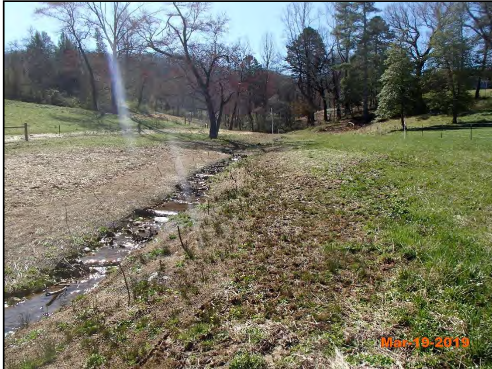
Coats Branch 1B – Permanent Photo Station 30 Looking Upstream
