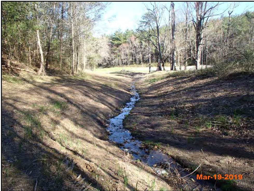
Raccoon Branch 1D – Permanent Photo Station 26 Looking Downstream
