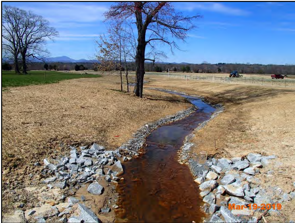
Fletcher Creek 2B – Permanent Photo Station 13 Looking Downstream from Crossing
