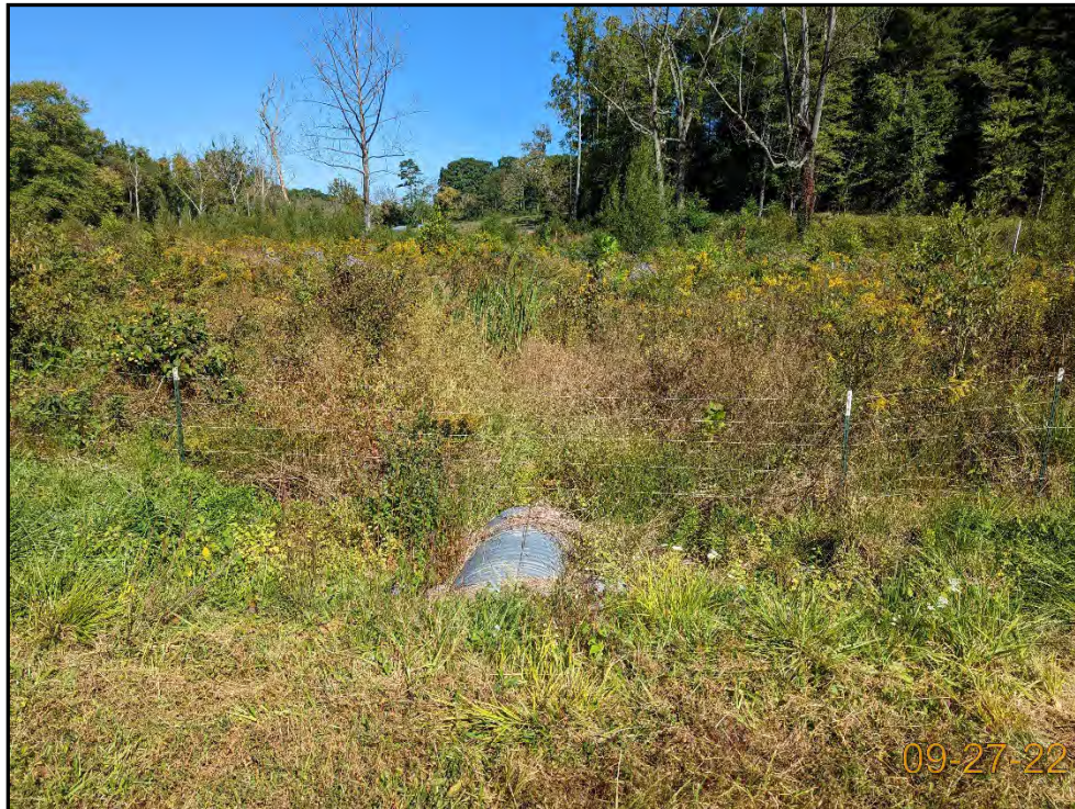
Coates Branch 1C – Permanent Photo Station 31 Looking Downstream from Crossing
