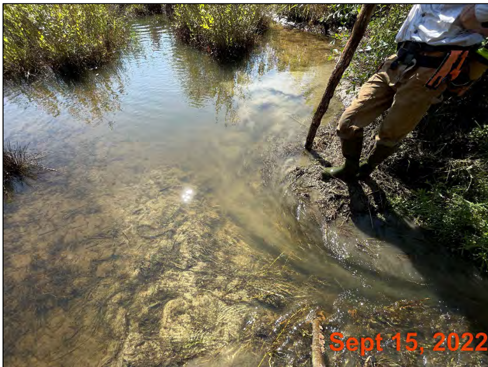
Breached Beaver Dam Weston Reach 1B, Station 424+50
