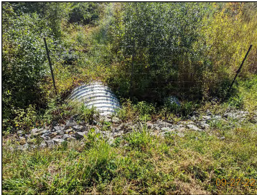
Fletcher Creek 1C – Permanent Photo Station 5 Looking Upstream from Crossing
