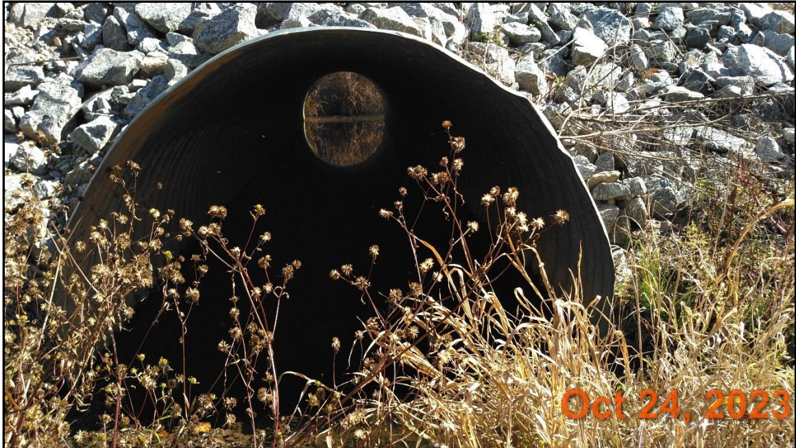
Fletcher Creek 2B – Permanent Photo Station 13 Looking Upstream through culvert.
