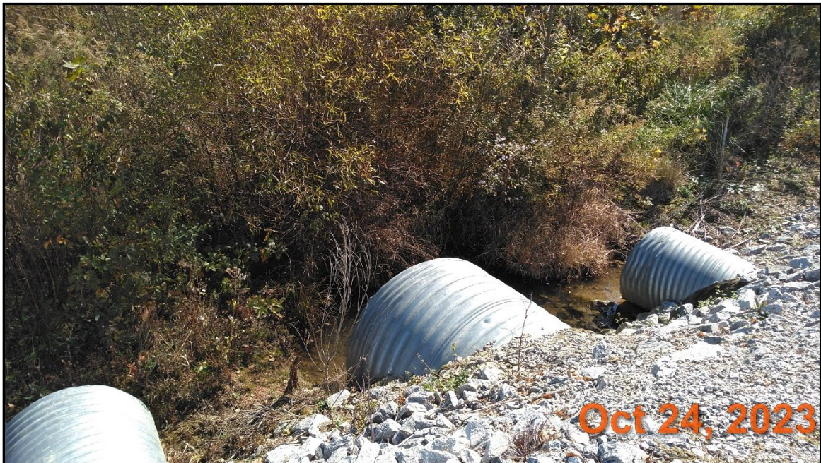
Fletcher Creek 2B – Permanent Photo Station 13 Looking Upstream from Crossing
