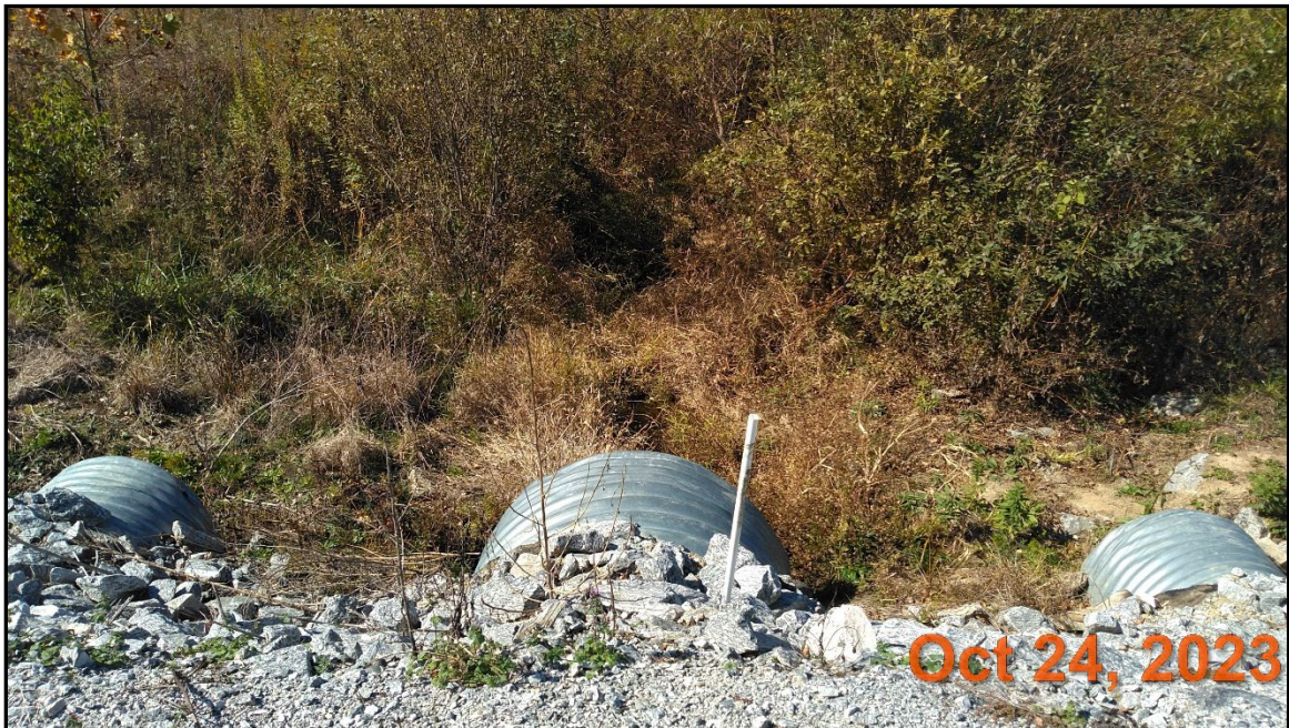
Fletcher Creek 2B – Permanent Photo Station 13 Looking Downstream from Crossing
