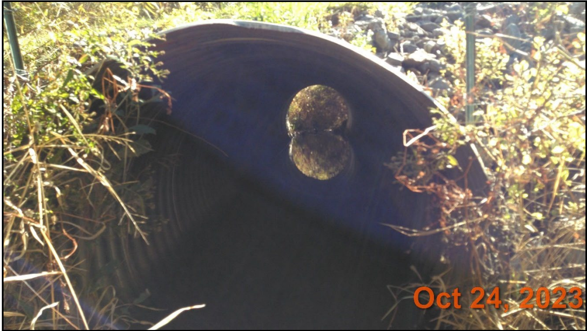
Fletcher Creek 1C – Permanent Photo Station 5 Looking upstream through culvert
