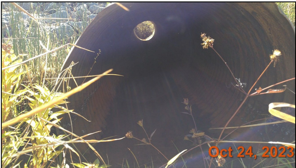
Coates Branch 1C – Permanent Photo Station 31 Looking Upstream through culvert.
