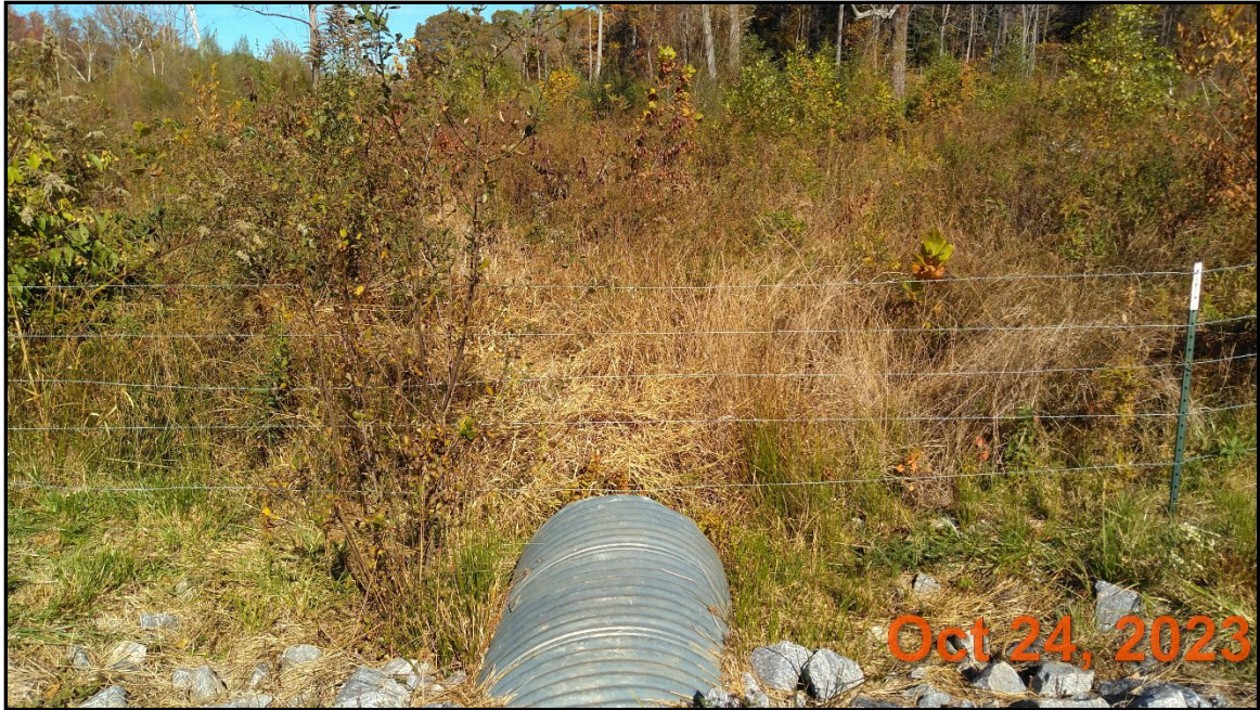
Coates Branch 1C – Permanent Photo Station 31 Looking Downstream from Crossing
