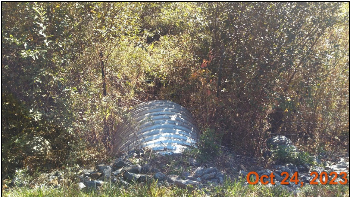
Fletcher Creek 1C – Permanent Photo Station 5 Looking Upstream from Crossing
