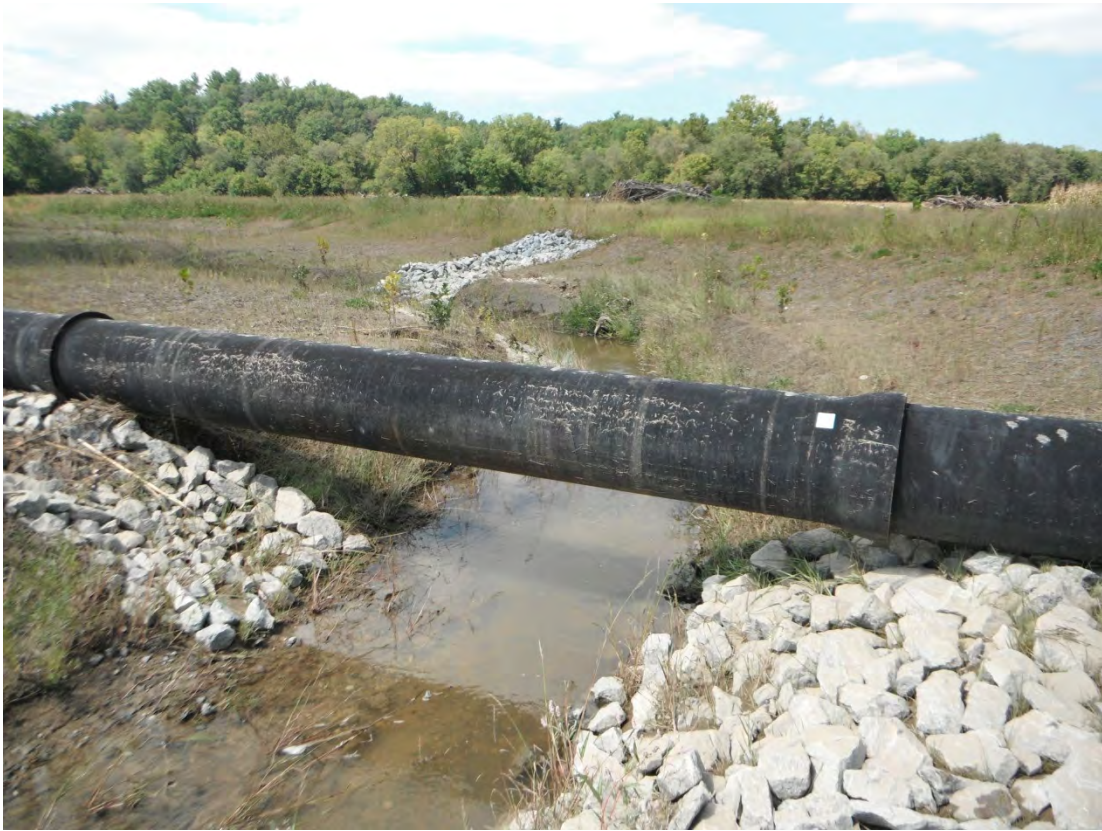
Lower Reach Photo Station 2 Downstream (9/16/2012 Year 0)
