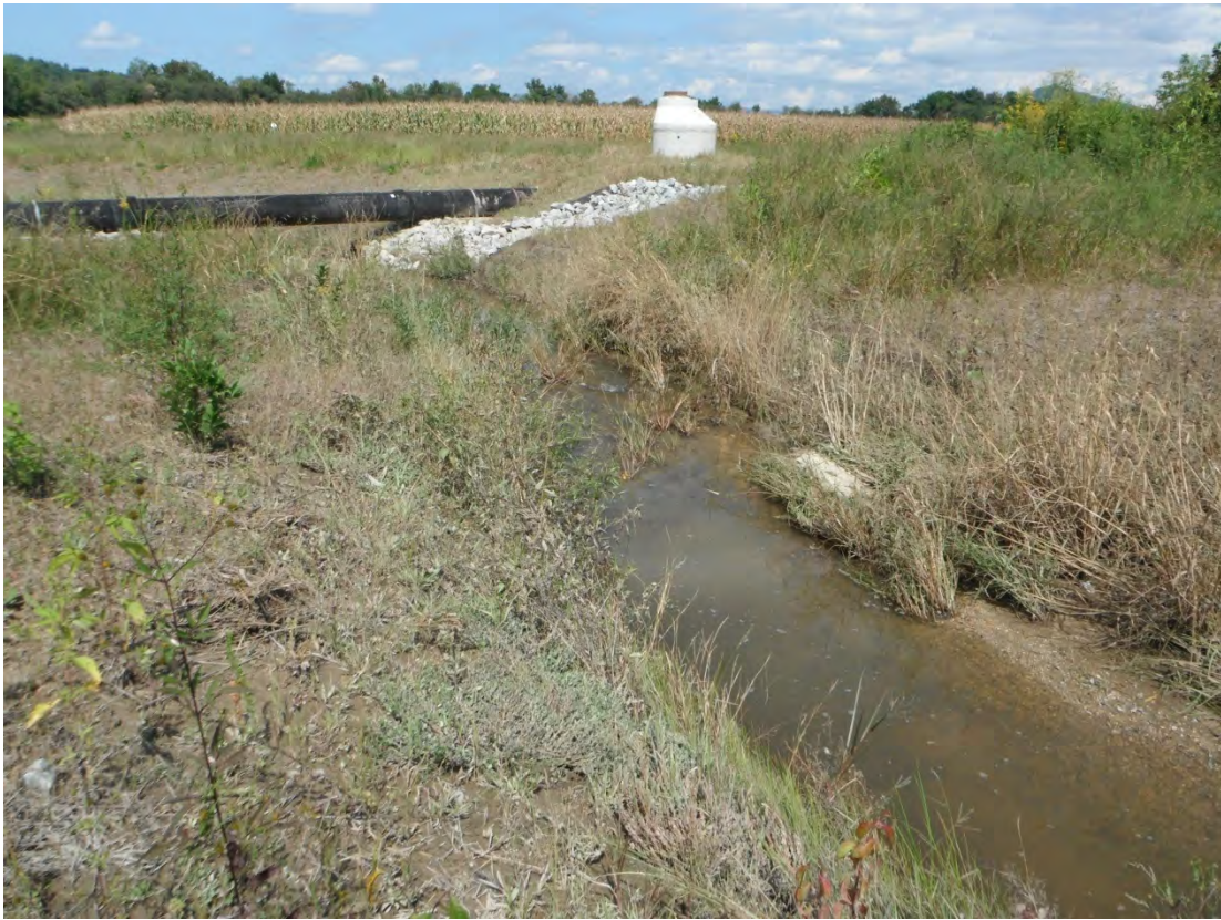
Lower Reach Photo Station 1 Downstream (9/16/2012 Year 0)
