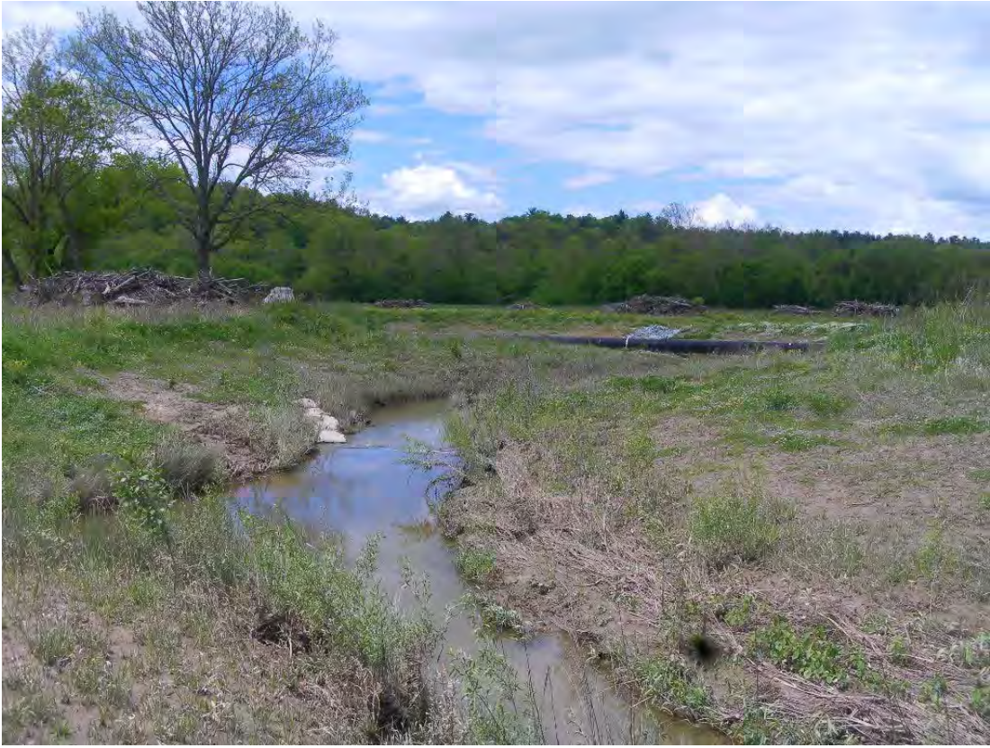
Upper Reach Photo Station 23 Downstream (5/7/2013 Year 1)
