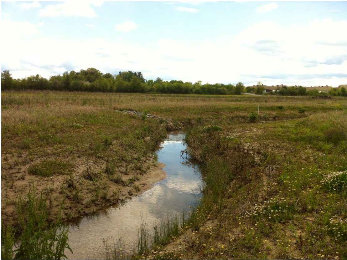
Upper Reach Photo Station 9 Downstream (5/7/2013 Year 1)
