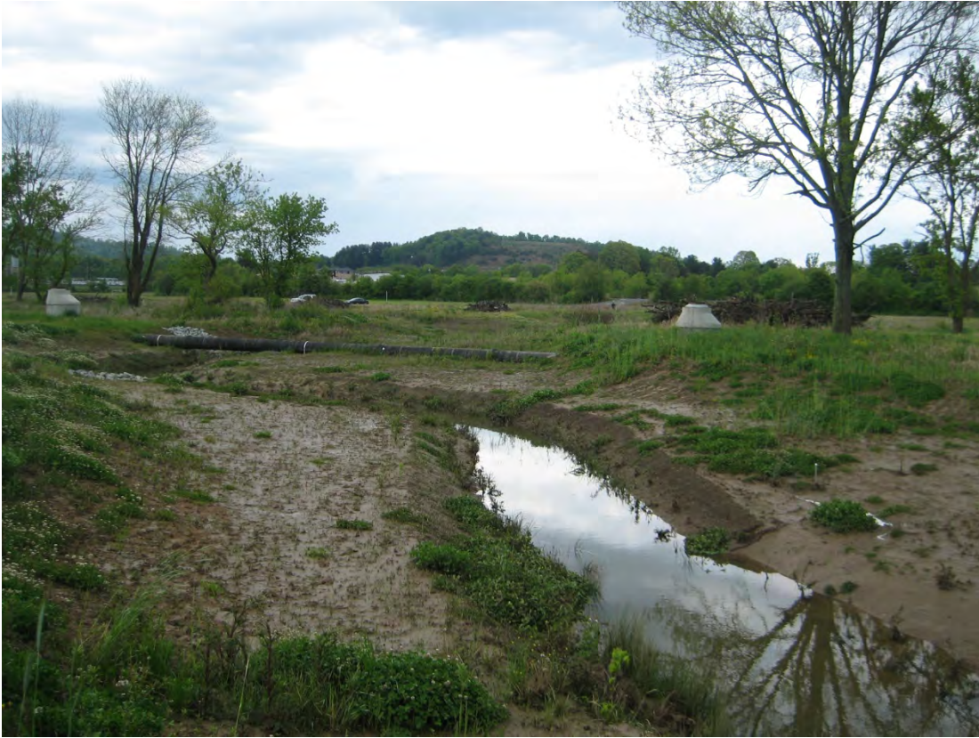
Lower Reach Photo Station 13 Downstream (5/08/2013 Year 1)
