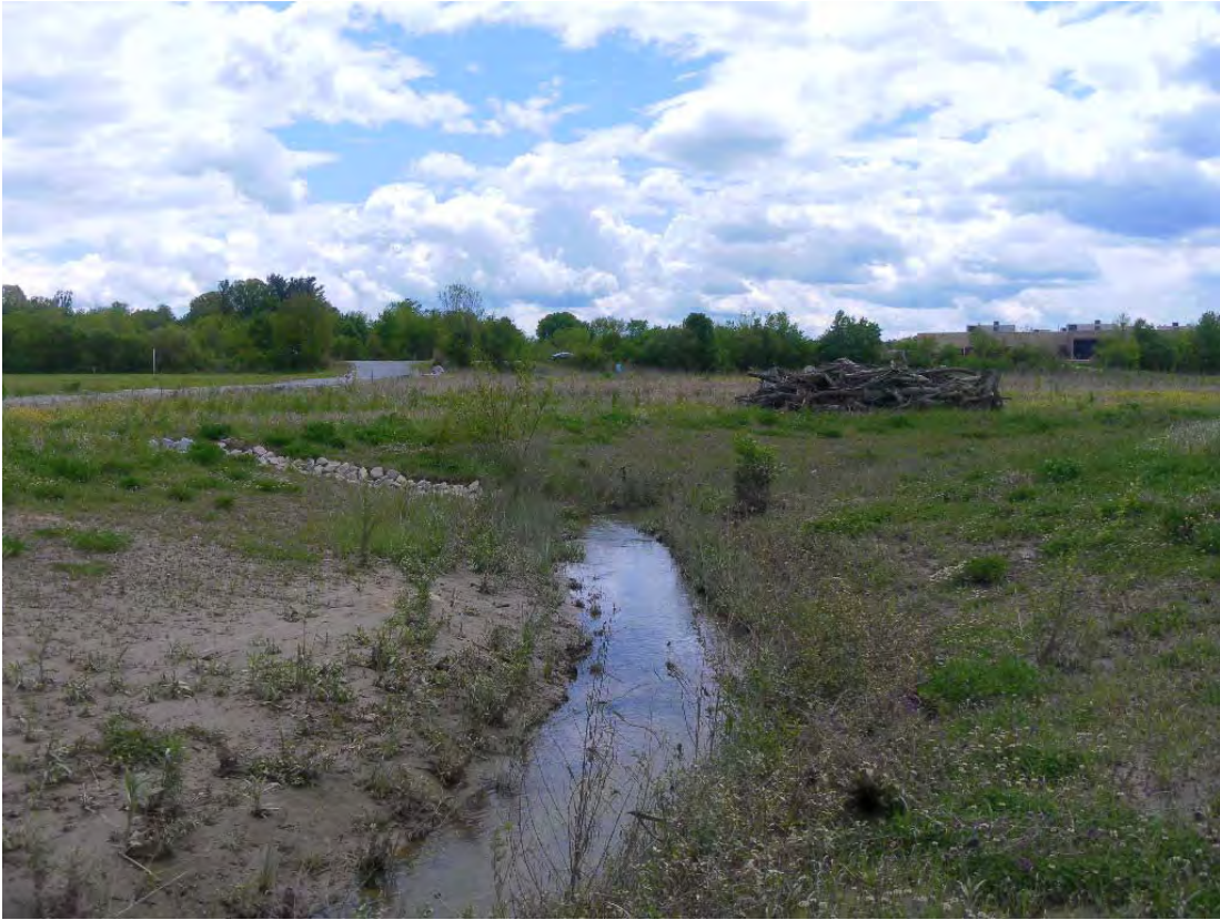
Upper Reach Photo Station 18 Downstream (5/7/2013 Year 1)
