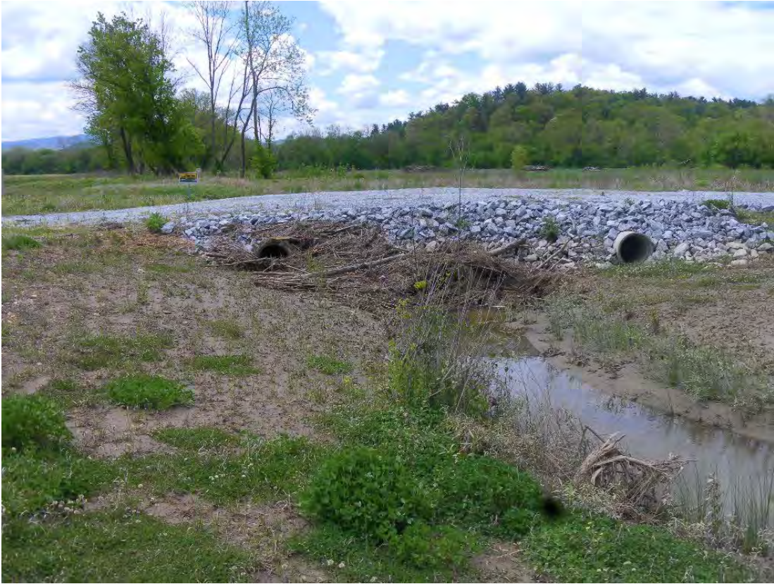
Upper Reach Photo Station 17 Downstream (5/7/2013 Year 1)
