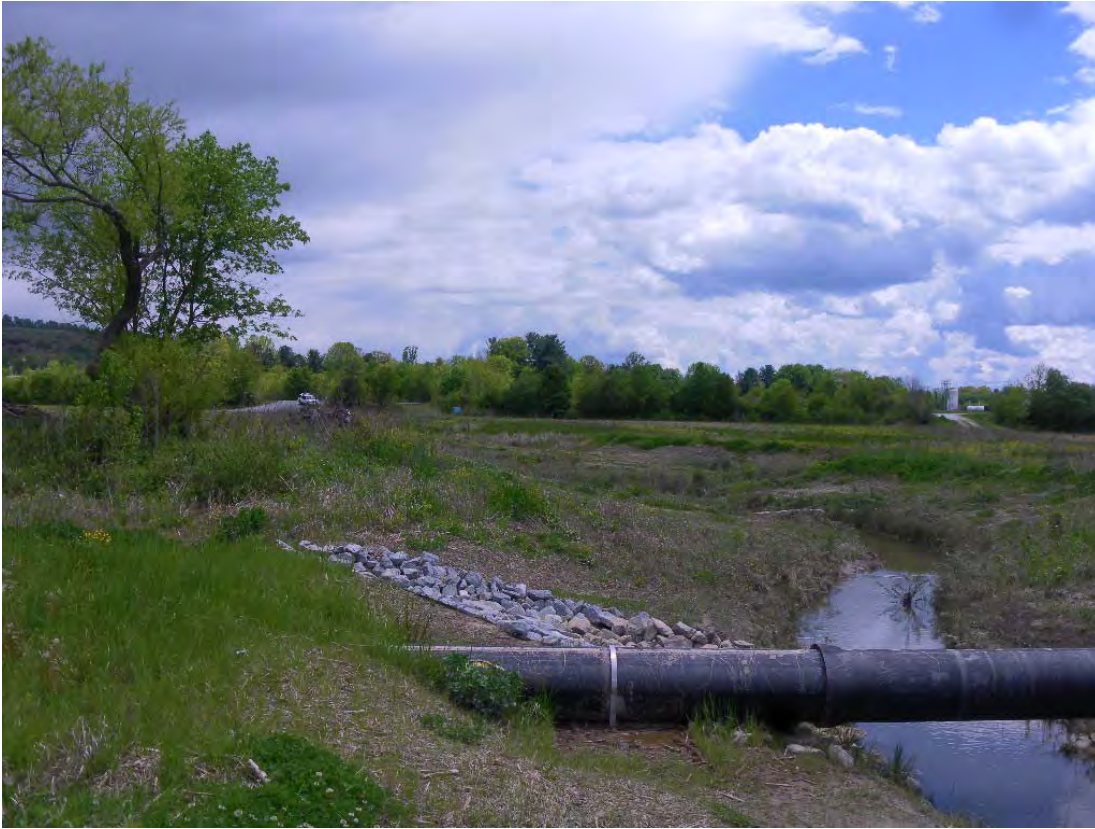
Lower Reach Photo Station 16 Downstream (5/07/2013 Year 1)
