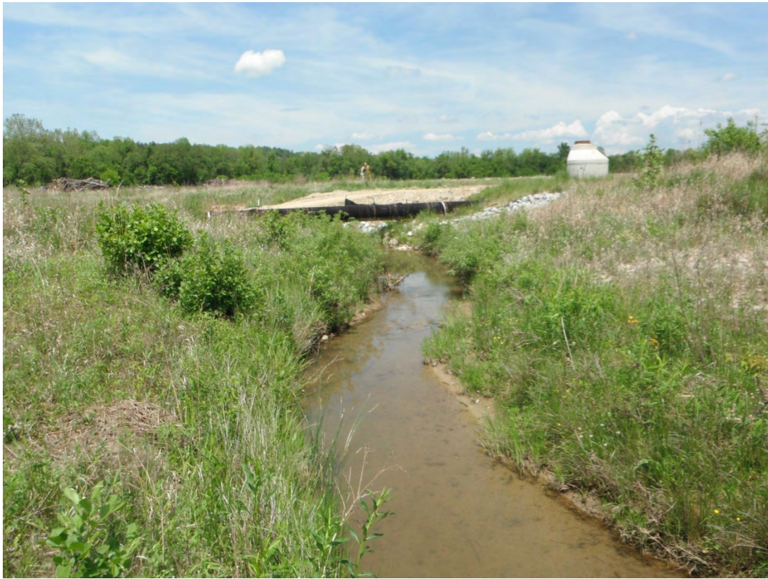
Lower Reach Photo Station 17 Downstream (5/12/2014 Year 2)
