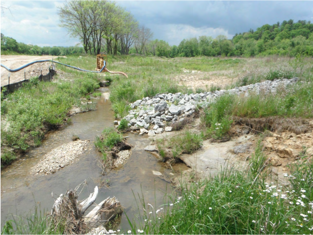
Lower Reach Photo Station 15 Downstream (5/12/2014 Year 2)
