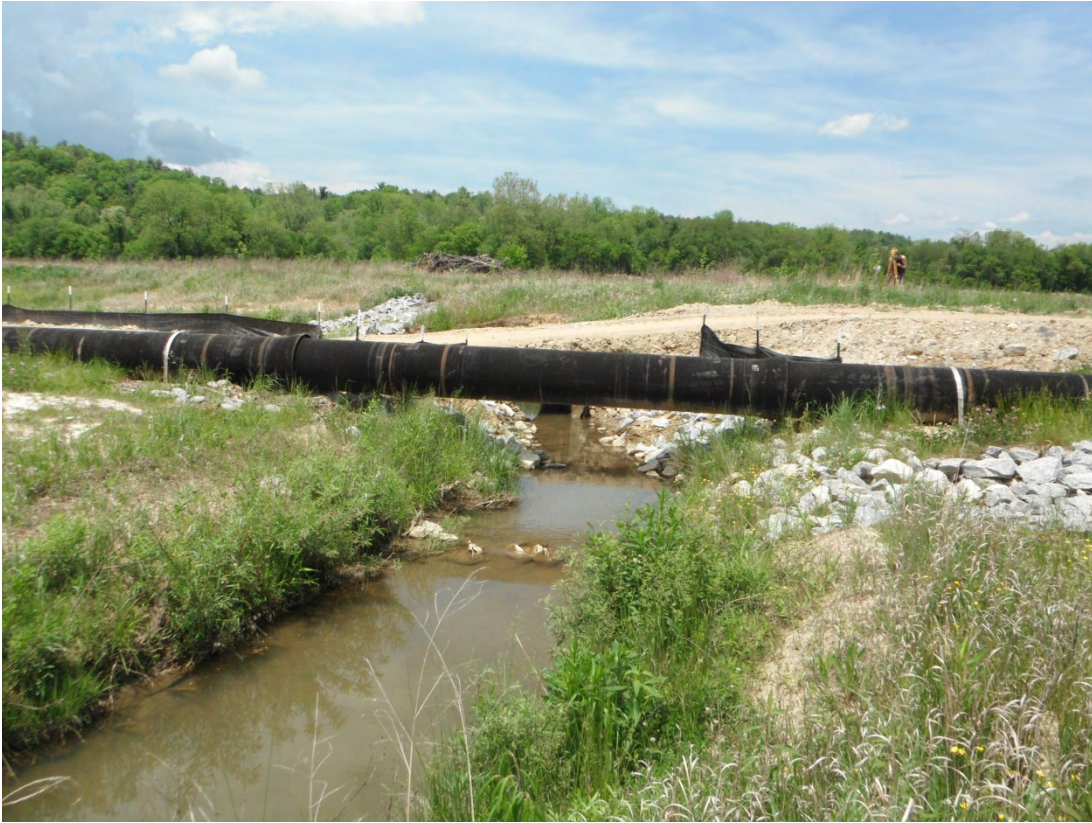
Lower Reach Photo Station 16 Downstream (5/12/2014 Year 2)
