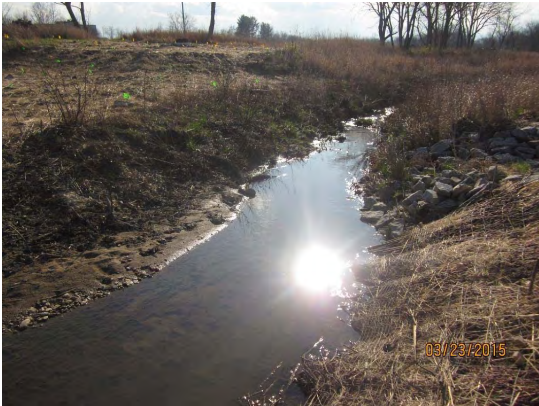
Lower Reach Photo Station 15 Downstream (3/23/2015 Year 3)
