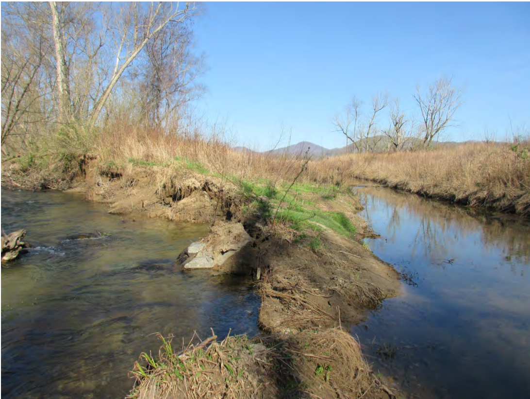
Looking upstream of Confluence with Cane Creek (3/22/2016 Year 4)
