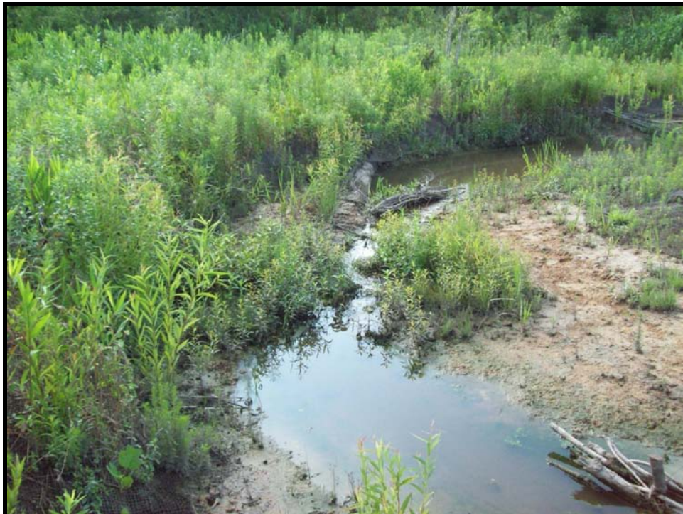
SPA4. Point bar at log vane; vegetation in channel.
