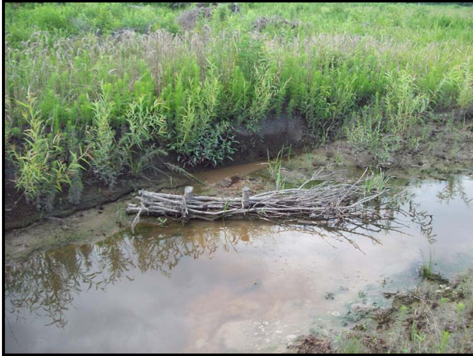
SPA3. Scour, erosion on left bank.
