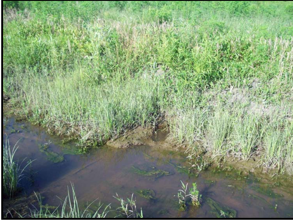
SPA5. Scour on right bank around bedded log structure.
