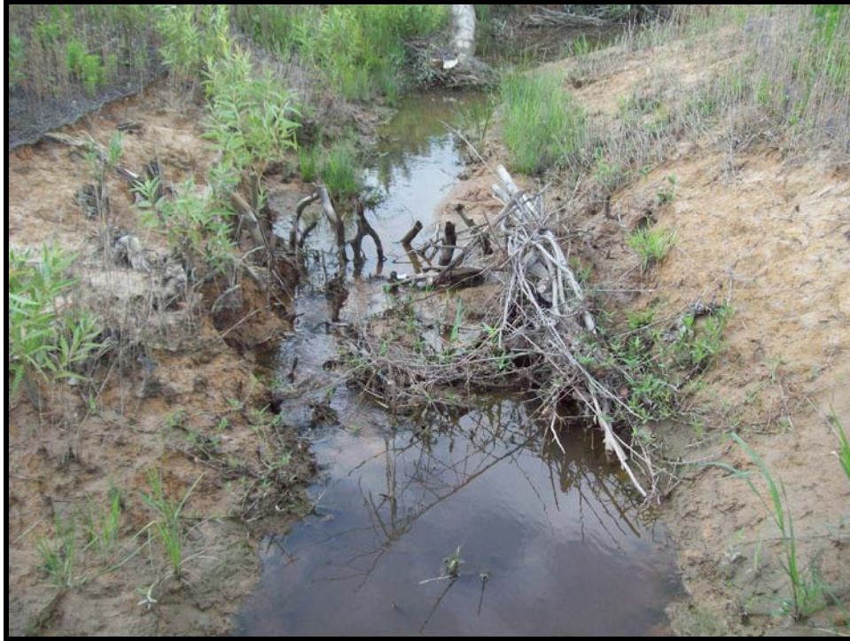
SPA1. Woody debris causing scour on left bank.
